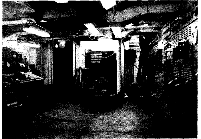
Figure 25.24 On-Board Electrical Outfit Zone
