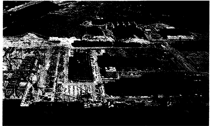
Figure 26.24 Samho Heavy Industries Shipyard in Korea Showing the Large Size and Space between Shops, Paint Halls and Building Dock
