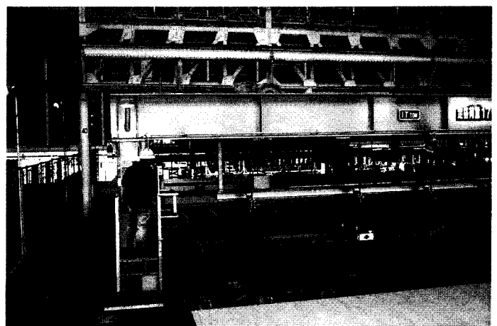
Figure 26.61 Steel Plate Conveying System
