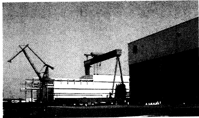
Figure 26.35 Typical Shipyard Buildings
