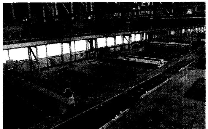
Figure 26.20 Typical Steel Shop (Panel Line)
