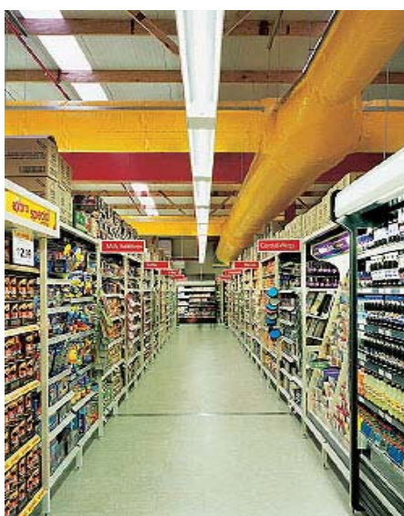
Figure 2.8 Suspended fabric air distribution ductwork for displacement ventilation (Coles Gisborne).
