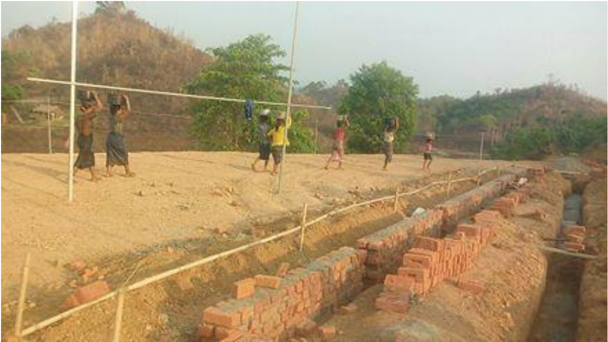
The construction process of the schools that Nay Myo Zin's organization built
