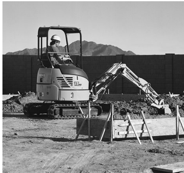
FIGURE 16.5 Footing excavation with a small backhoe. (Courtesy of John Deere, Moline, Illinois)
