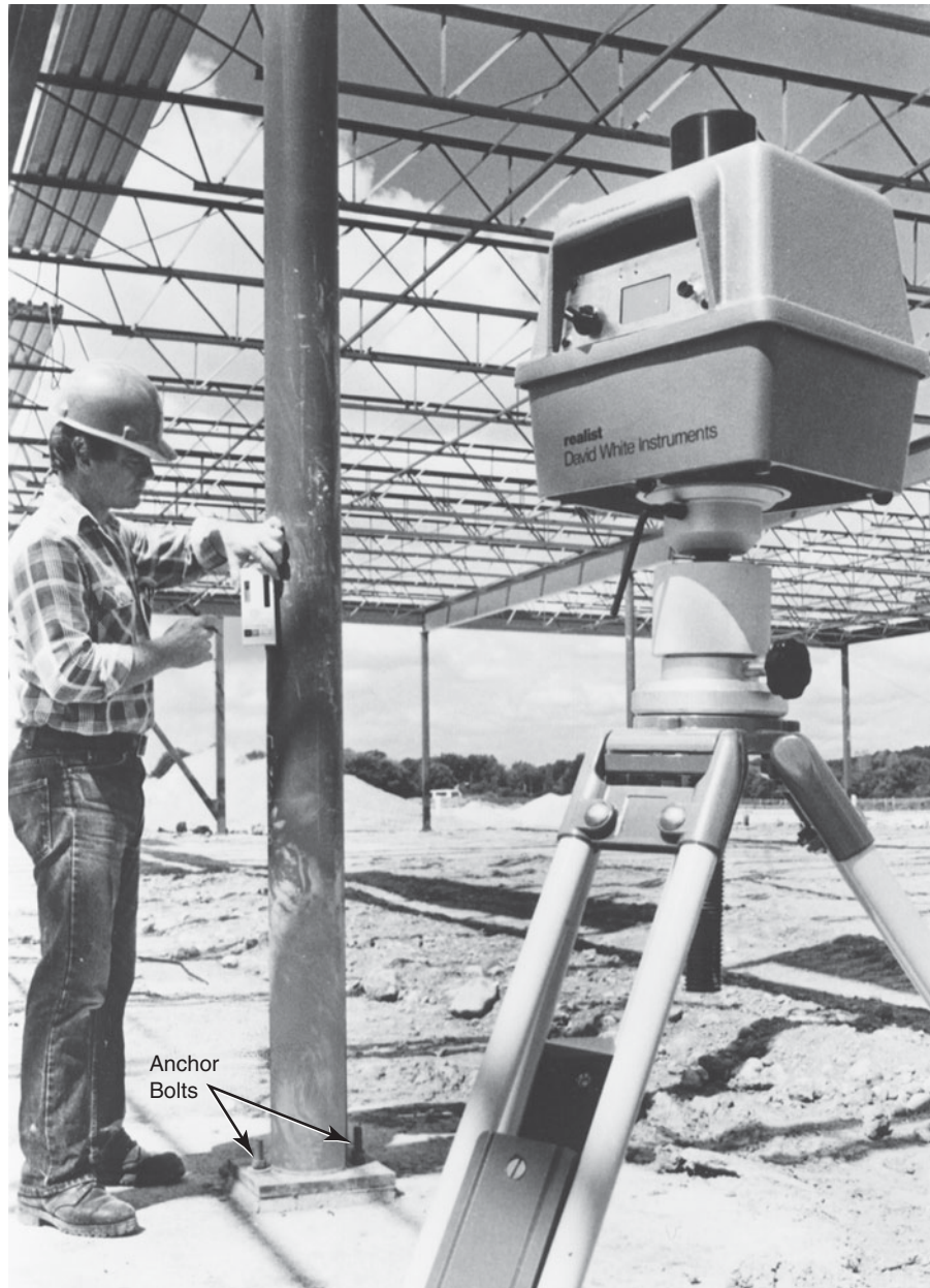
FIGURE 16.9 Electronic level. (a) Marking vertical control (4-ft marks on a steel column); (continued)
