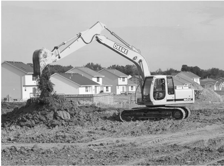
FIGURE 16.4 Excavation for house basement and footings. (Courtesy of John Deere, Moline, Illinois)
