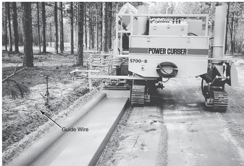
FIGURE 13.6 Slip-form concrete paver: line and grade are provided by string line (can also be guided by laser). Precision of \frac{1}{8} in. or 0.01 ft. (Courtesy of Ausran)
