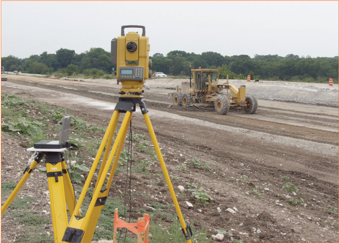
Total station guidance and control. A hybrid Topcon total station tracks a motor grader equipped with a Topcon 3D-LPS automatic control system. This local position system (LPS) uploads plan information directly from the attached field computer and relays the elevation and slope data via a laser beam emitted from the total station. This system permits high-speed automatic grading to an accuracy of a few millimeters. (Courtesy of Topcon Positioning Systems, Inc., Pleasanton, Calif.)
