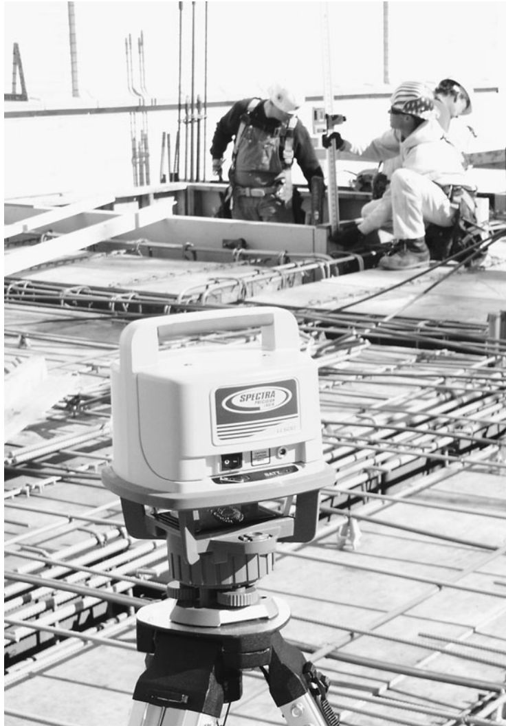
FIGURE 16.10 Spectra precision rotating laser level and an electronic receiver being used to set concrete forms to the correct elevation. (Courtesy of Trimble)
