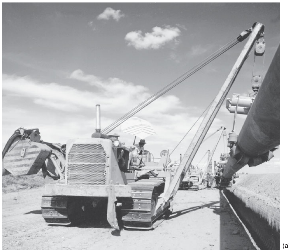
FIGURE 14.2 (a) Pipeline installation. (Courtesy of Caterpillar, Inc.)
