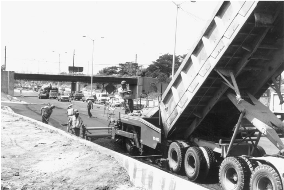
FIGURE 13.9 Asphalt spreader laying asphalt to finished grade as marked on the curb face. (Courtesy of Caterpillar Inc., Peoria, Illinois)
