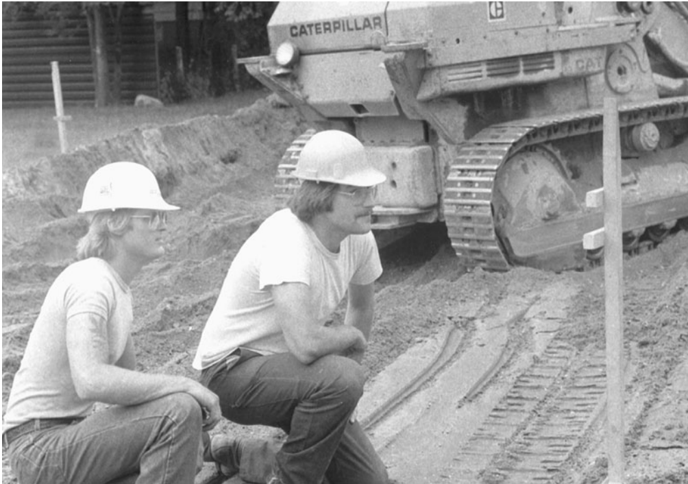
FIGURE 13.7 Progress of street construction being monitored by the use of sight rails (batter boards).
