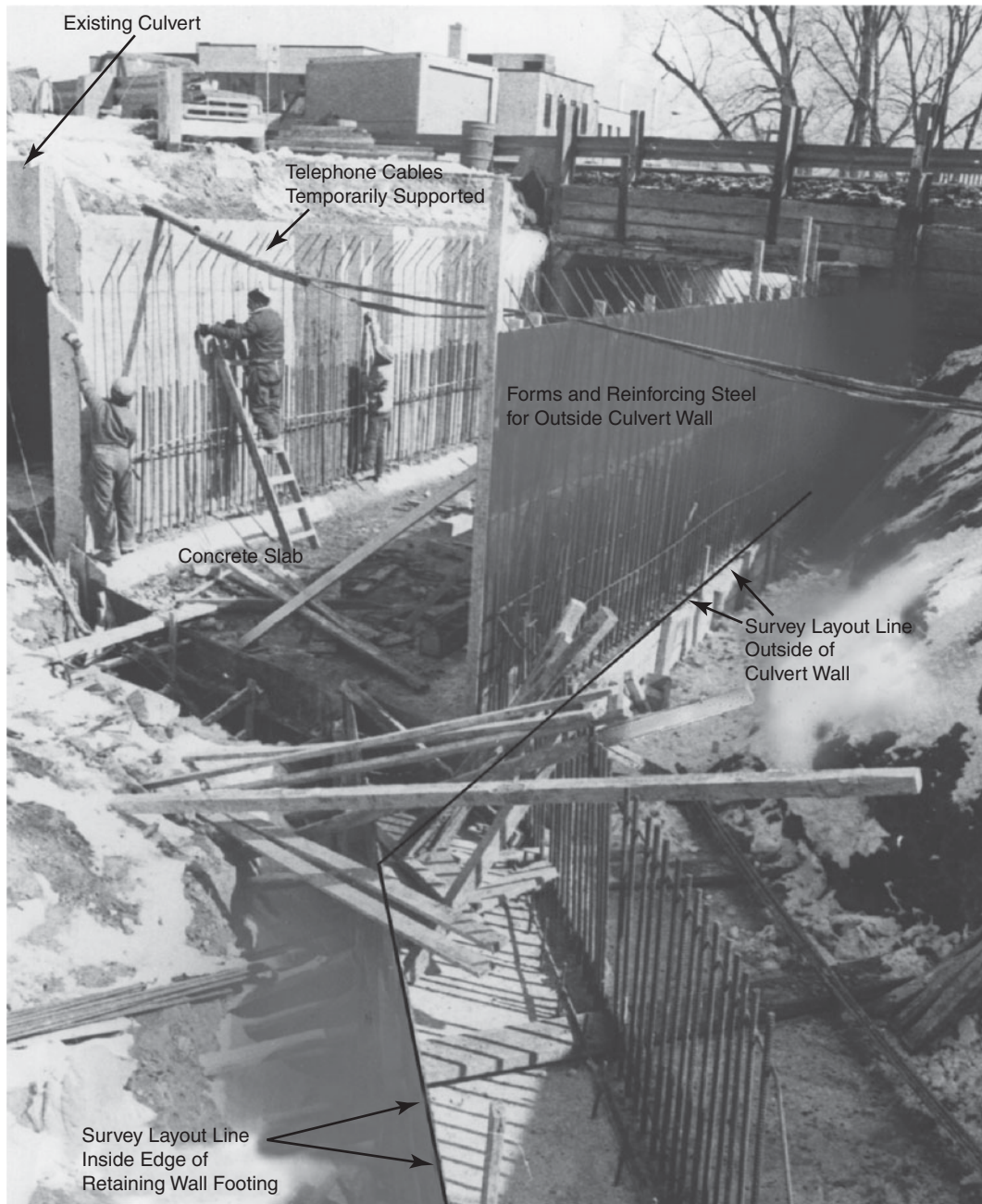
FIGURE 15.4 Concrete culvert construction addition, showing floor slab, wing wall footing, and culvert walls—with reinforcing steel and forms.
