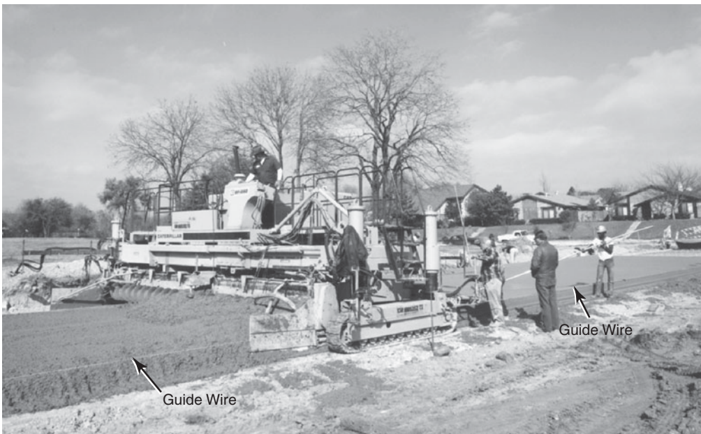
FIGURE 13.8 Concrete paver, controlled for line and grade by guide wires established from grade stakes supplied by the surveyor. (Courtesy of Caterpillar, Inc., Peoria, Illinois)
