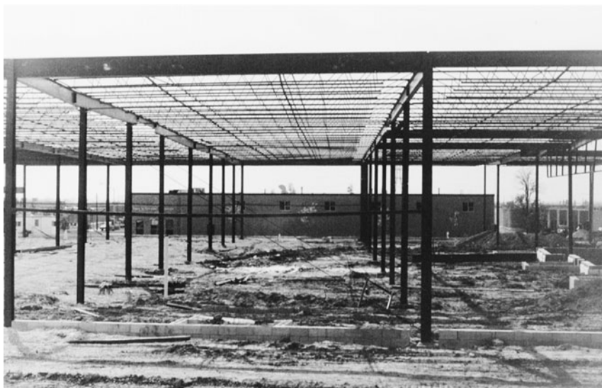
FIGURE 16.6 Single-story building columns and column footings.
