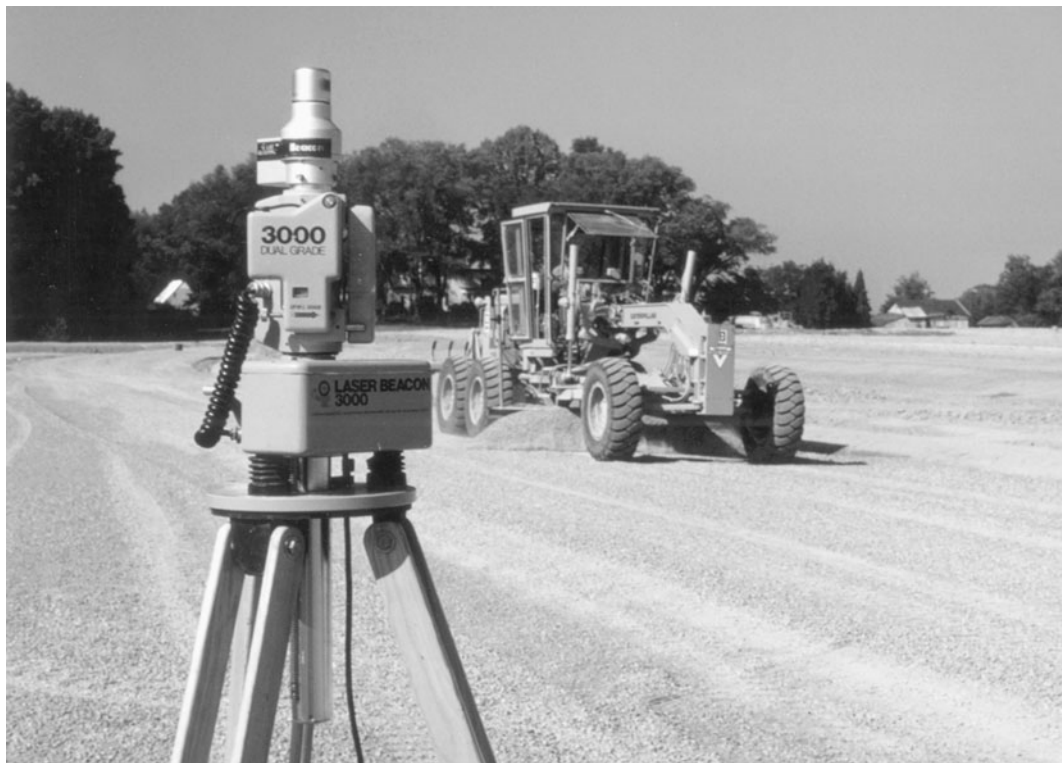
FIGURE 12.18 Rotating laser shown controlling fine grading operations by a road grader. (Courtesy of Leica Geosystems Inc.)
