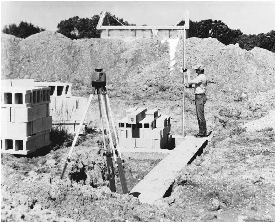
FIGURE 16.12 Autolaser 300, shown checking the footing elevations prior to construction of the concrete-block walls. (Courtesy of CST/Berger-David White)
