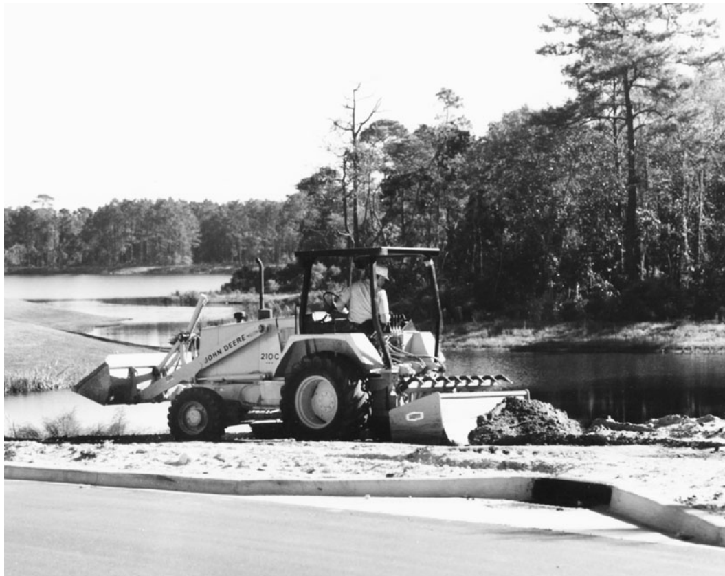
FIGURE 13.16 Fine grading by landscaping/pulverizing attachment on loader. (Courtesy of John Deere, Moline, Illinois)
