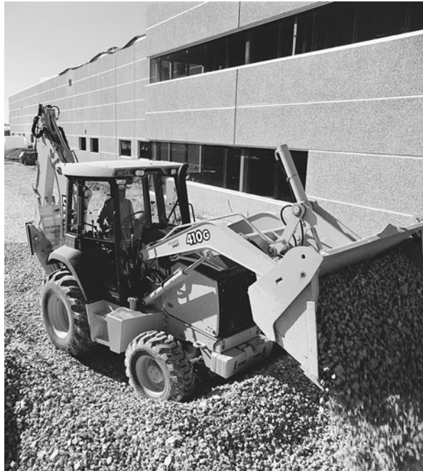
FIGURE 13.15 Rough grading by loader/backhoe. (Courtesy of John Deere, Moline, Illinois)
