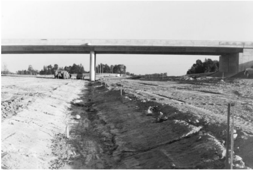
FIGURE 12.22 A multilane divided highway, showing center drainage with grade stakes.
