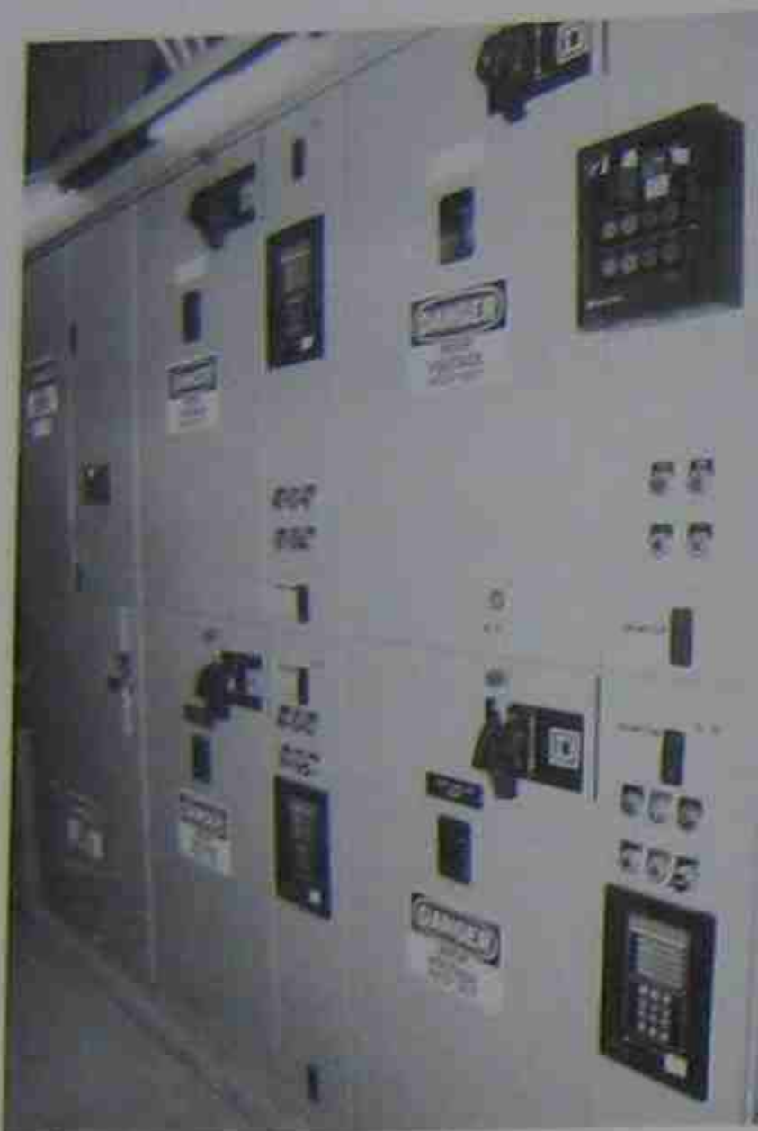
Figure 31.20 This 600-V, 3-phase motor control center is equipped with PowerLogic ® devices that provide sophisticated monitoring capabilities such as active and reactive power, voltage, current, and waveform analysis. It includes Internet transmission capabilities and possesses embedded Web pages. (Courtesy of Schneider Electric)
