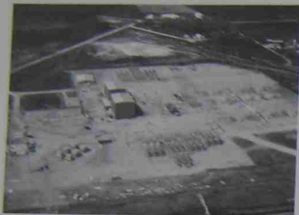
Figure 28.21c Aerial view of the Coal Creek Terminal showing the two valve halls that respectively produce the +400 kV and -400 kV dc voltage. The switchyard contains circuit breakers, transformers, and filters. (Courtesy of United Power Association)
