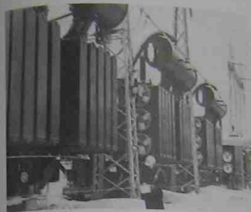
Figure 28.14 Three-phase converter transformer bank rated 230 kV/127 kV/17 kV composed of 3 single-phase transformers each rated 323 MVA. (Courtesy of Manitoba Hydro)
