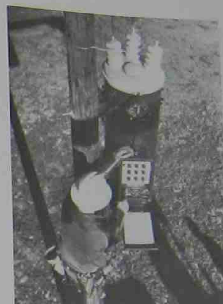
Figure 26.29 Automatic tap-changing autotransformer maintains steady voltages on long rural lines. (Courtesy of General Electric)
