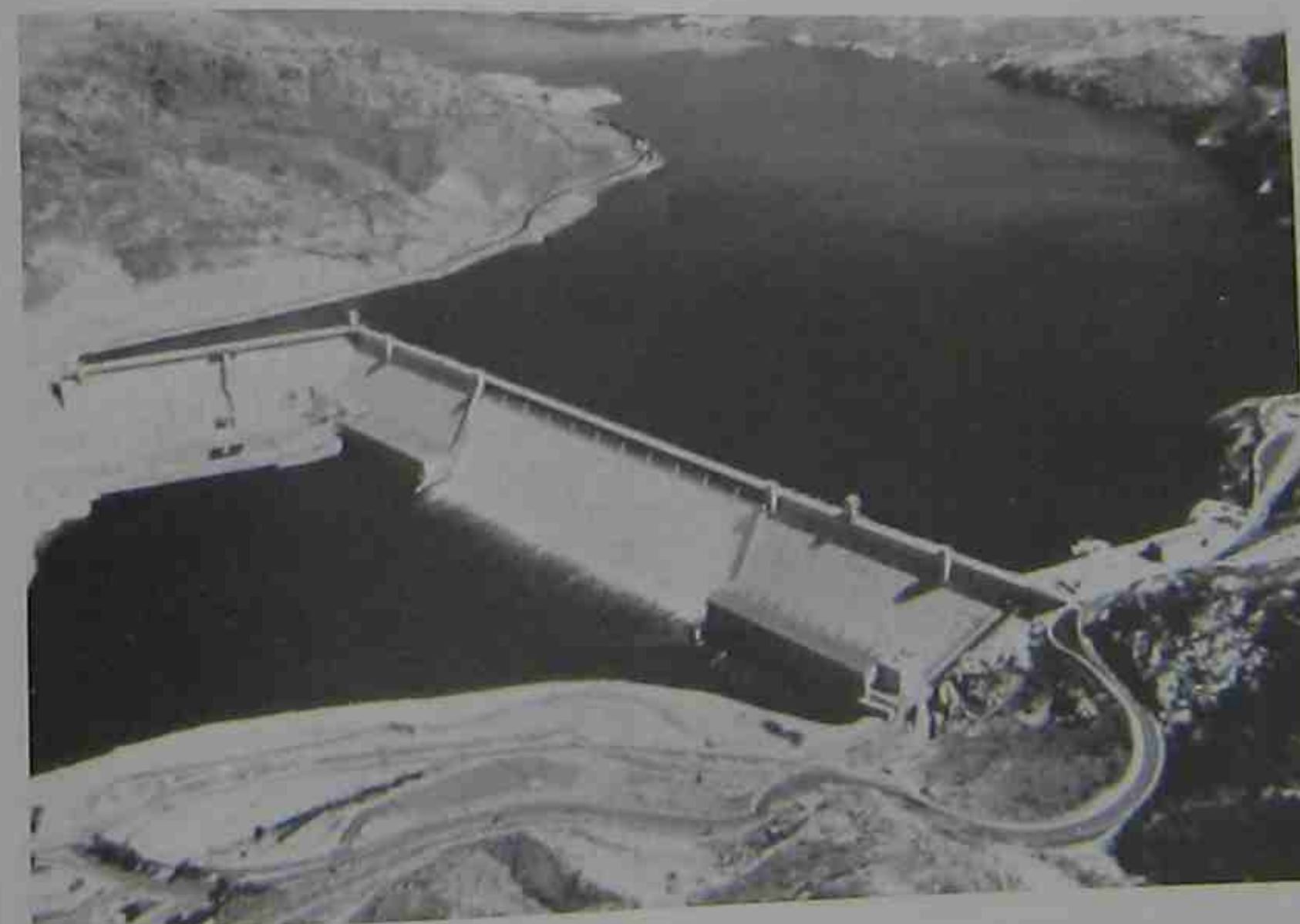
Figure 24.8 The Grand Coulee Dam on the Columbia River in the state of Washington is 108 m high and 1270 m wide. It is the largest hydropower plant in the world, having 18 generating units of 125 MW each and 12 generating units of 600 MW each, for a total of 9450 MW of installed capacity. The spillway can be seen in the middle of the dam. (Courtesy of General Electric)
