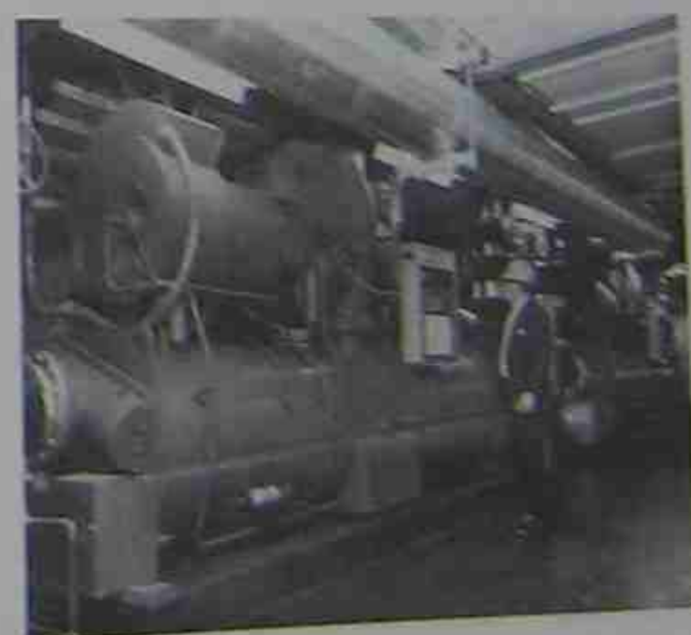
Figure 28.17 Partial view of the refrigeration unit needed to cool the inverters. (Courtesy of Manitoba Hydro)
