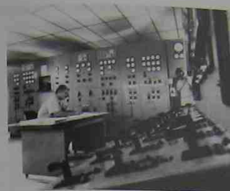
Figure 24.7 Technicians in the control rooms of two generating stations communicate with each other, or with a central dispatching office, while supervising the operation of their respective generating units.
