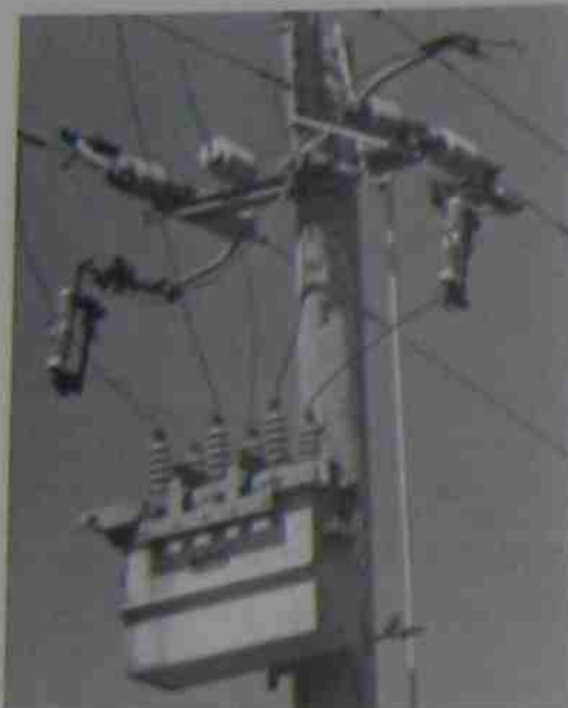
Figure 26.33 Automatic recloser protecting a 3-phase feeder.
