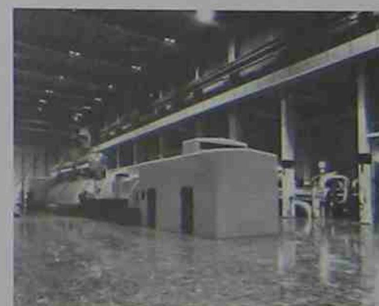
Figure 24.22 This 540 MW steam-turbine generator set runs at 3600 r/min, generating a frequency of 60 Hz. The low-pressure turbine and alternator are in the background. (Courtesy of General Electric)
