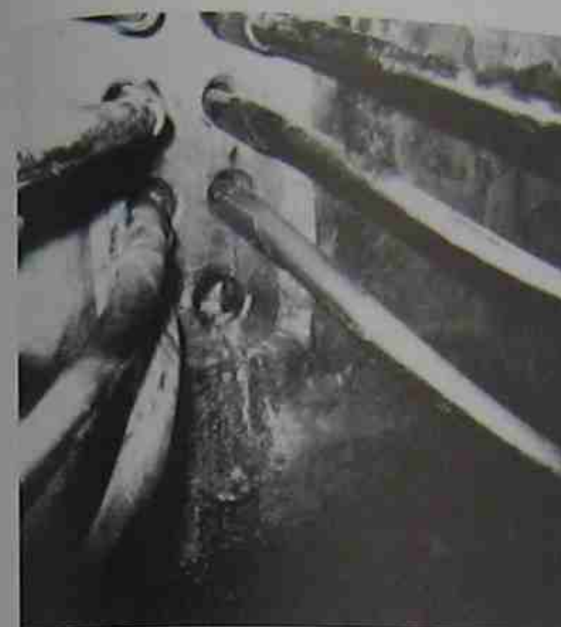
Figure 26.27 MV underground feeders in concrete duct.
