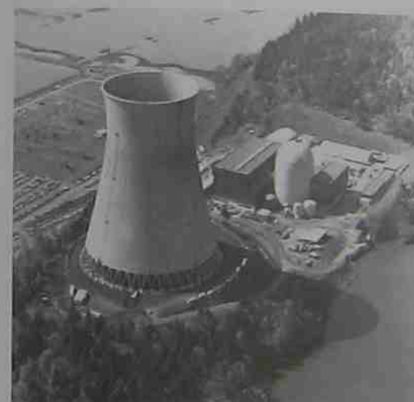
Figure 24.21 Cooling tower installed in a nuclear power station in Oregon. The generator output is a 1280 MVA at a power factor of 0.88. Tower characteristics: height: 152 m; diameter at the base: 117 m; diameter at the top: 76 m; cooling water: 27\text{ m}^3/\text{s} ; water loss by evaporation: 0.7\text{ m}^3/\text{s} . The temperature of the cooling water drops from 44.5^{\circ} to 24^{\circ} as it passes through the tower. (Courtesy of Portland General Electric Company)
