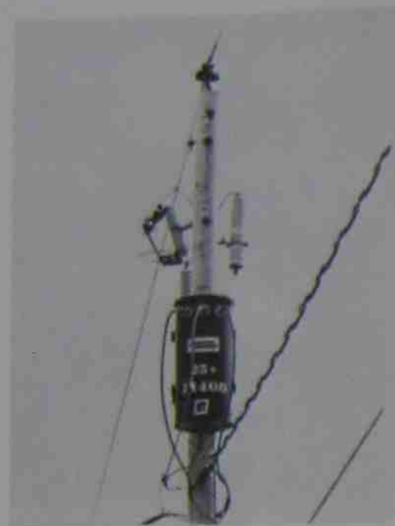
Figure 26.30 A fused cutout (top left) and lightning arrester (top right) protect a single-phase transformer rated 25 kVA, 14.4 kV/240 V–120 V, 60 Hz.
