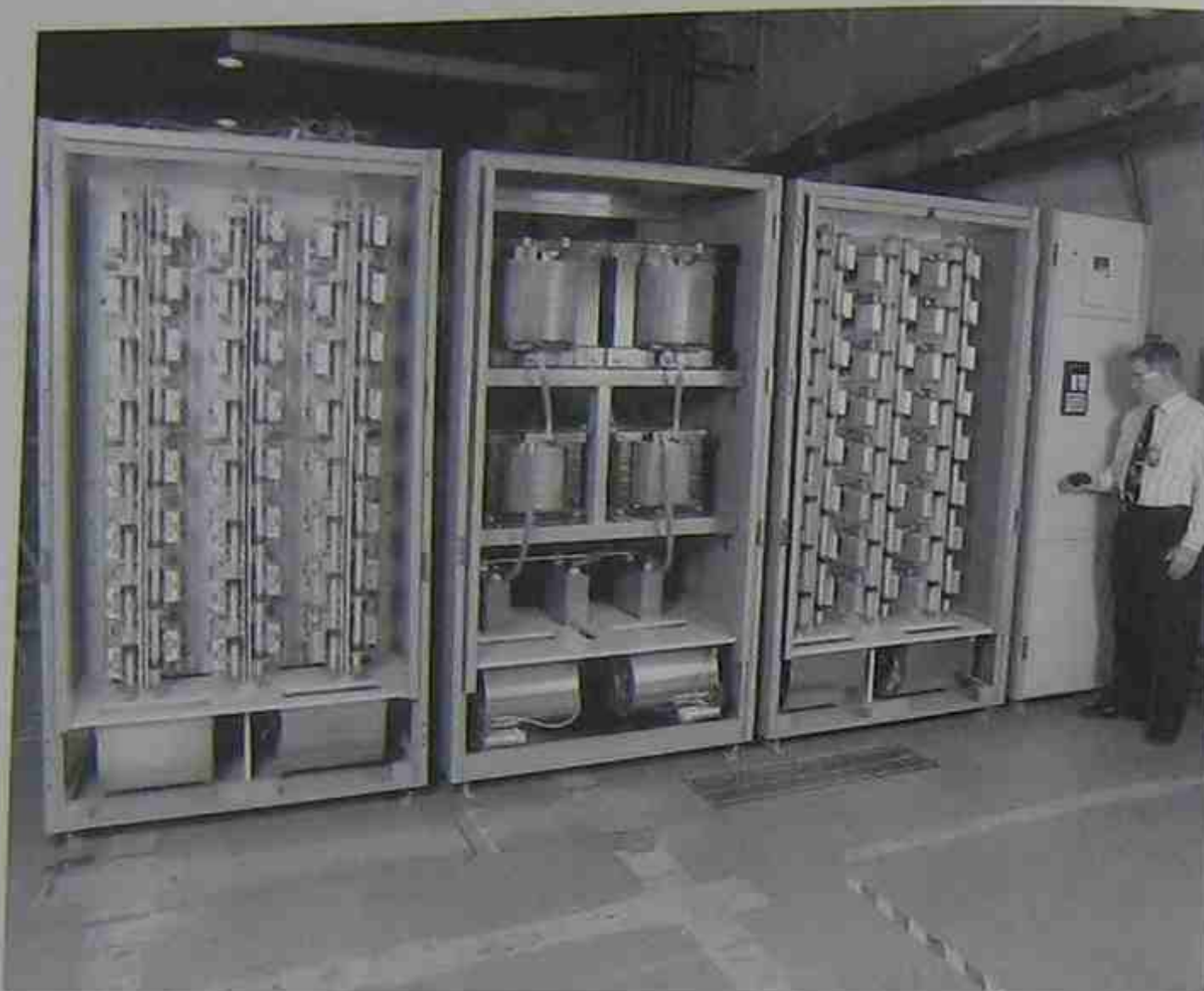
Figure 29.32 This \pm 2 MVA converter assembly can be used in either a shunt or series compensator (DSTATCON or DVR). (Courtesy of Westinghouse Electric Corporation)
