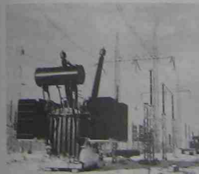
Figure 28.15 View of one 0.5 H smoothing inductor on the 450 kV dc side of the inverter station. The second inductor can be seen in the distance (lower right-hand corner). The space between the two units permits installing the filters on the dc side. (Courtesy of Manitoba Hydro)
