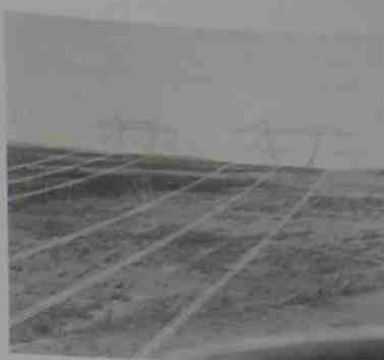
Figure 25.34 Two 735 kV transmission lines in parallel carrying electrical energy to a large city. Each phase is composed of 4 bundled conductors (see Fig. 25.7). (Courtesy of Hydro-Québec)
