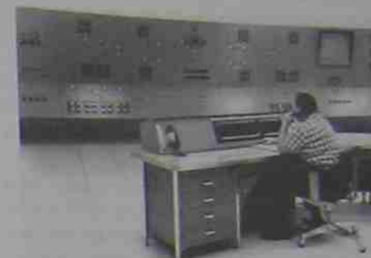
Figure 24.7 Technicians in the control rooms of two generating stations communicate with each other, or with a central dispatching office, while supervising the operation of their respective generating units.
