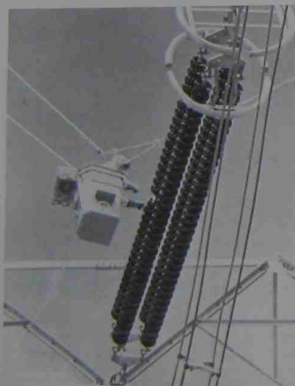
Figure 25.4 Lineman working bare-handed on a 735 kV line. He is wearing a special conductive suit so that his body is not subjected to high differences of potential. In the position shown, his potential with respect to ground is about 200 kV. (Courtesy of Hydro-Québec)
