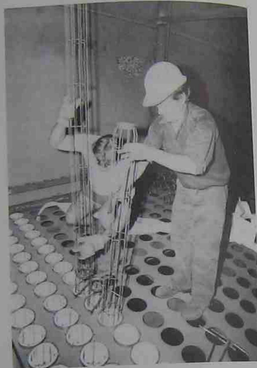
Figure 24.27 Installation of the fabric filter bags. Each bag is 15 m long and 16 cm in diameter. (Courtesy of Electricity Commission of New South Wales)
