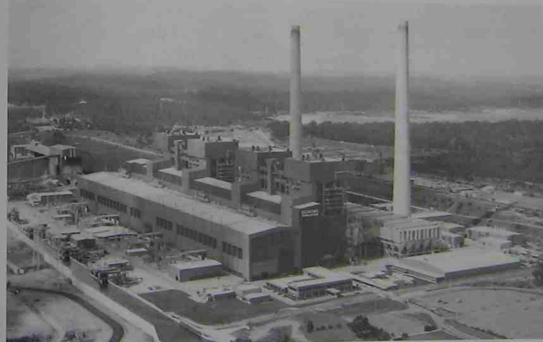
Figure 24.25 View of the Eraring Power Station in Newcastle, Australia. The large building on the left is the turbine-generator hall: 27 m wide \times 38 m high \times 418 m long. To the right can be seen the four structures that house the steam boilers. A portion of the flue gas cleaning system can be seen between the emission stack in the foreground and the boiler structures. (Courtesy of the Electricity Commission of New South Wales)
