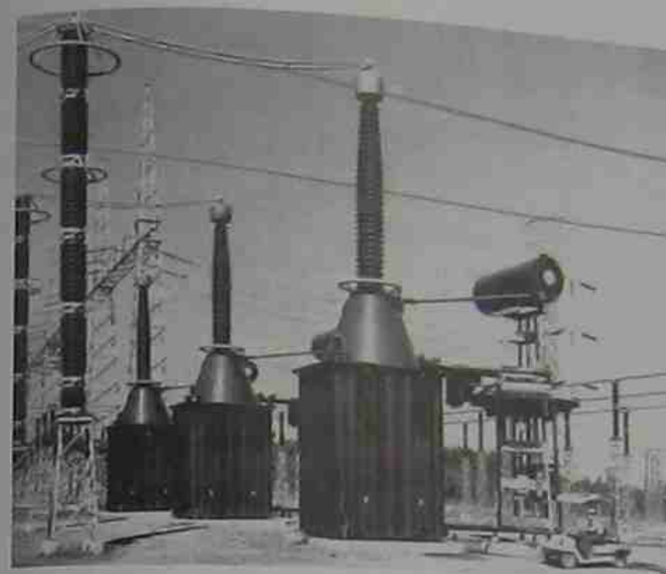
Figure 25.37 Three large 110 Mvar, single-phase reactors installed in a substation to compensate the line capacitance of a very long 3-phase 735 kV transmission line. (Courtesy of Hydro-Québec)
