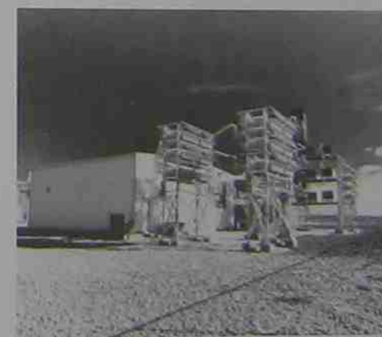
Figure 25.39 Static var compensator for HV line. (Courtesy of General Electric)
