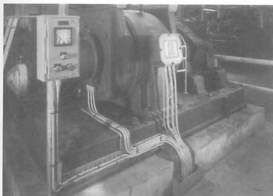
Fig. 10.4(b) Wiring to a motor MM CABLES PYROTENAX
