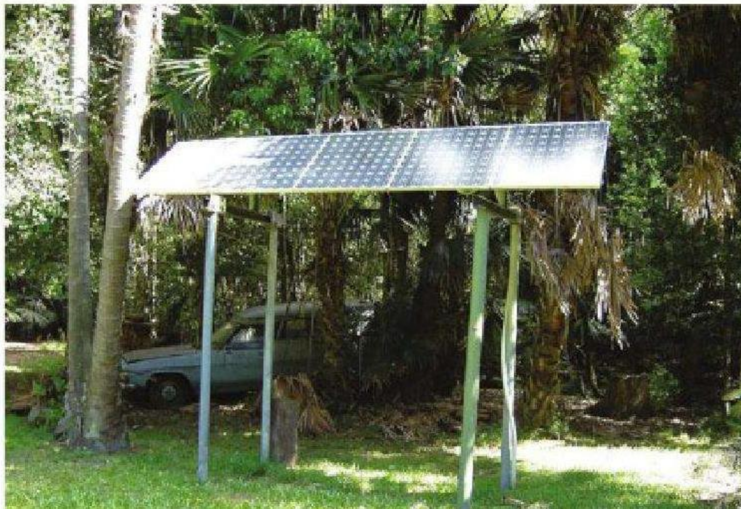
Figure 7.4 Poorly chosen site where trees are shading the PV array
