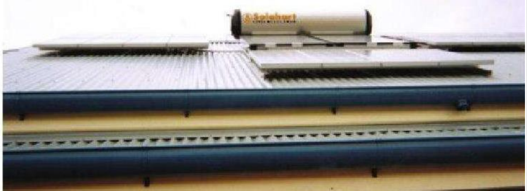
Figure 6.1 This mounting scheme allows good ventilation. Mounting panels closer to the roof increases operating temperature and thereby lowers system performance
