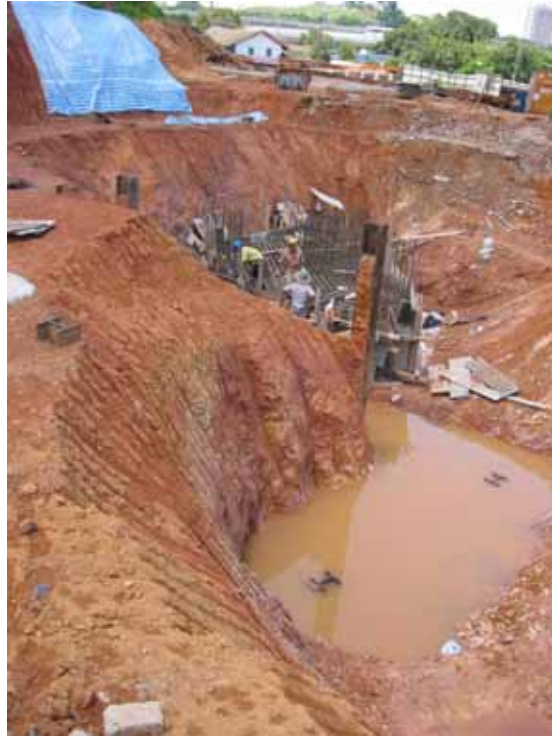
Figure 85: Too steep temporary cut slope
