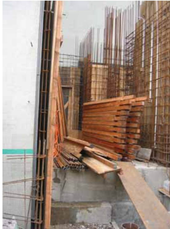
Figure 77: Reinforcement for wall before formwork erection
