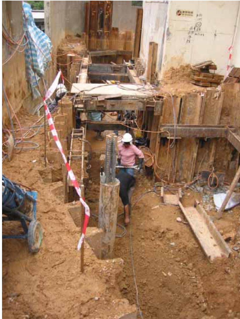
Figure 84: Excavation works at 2 nd layer before the 1 st layer strut completed In general, the above irregularity is very common for a small construction site because the following reasons:
