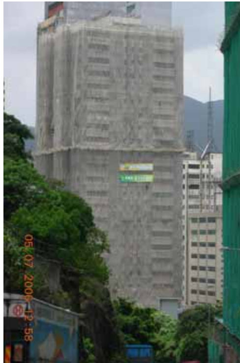
Figure 36: Bamboo scaffolding is used as working platform in renovation works Renovation
