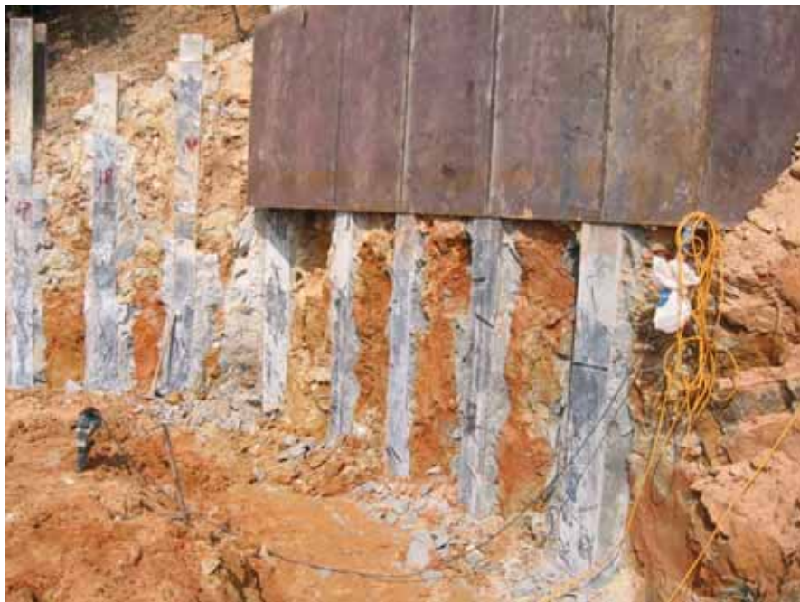
Figure 81: Soldier Pile and Lagging wall were used in excavation
