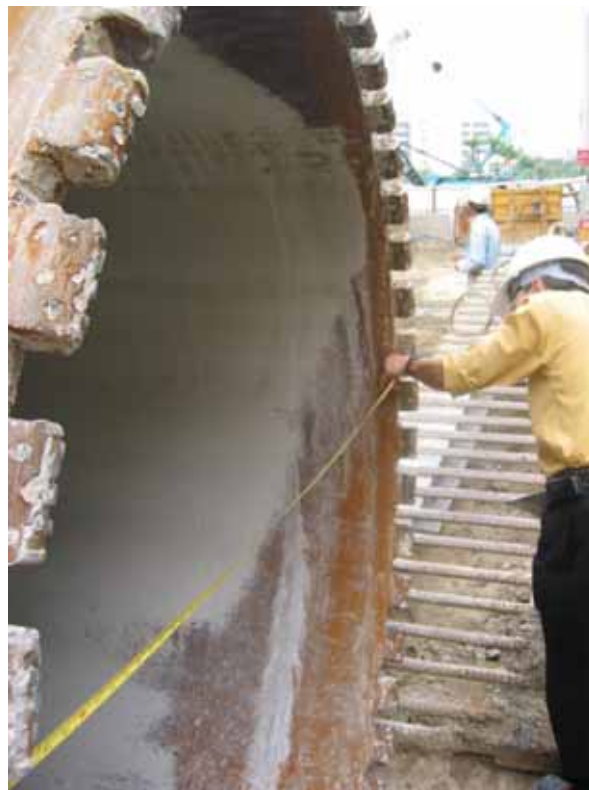
Figure 11: Engineer check the diameter of steel casting before drilling
