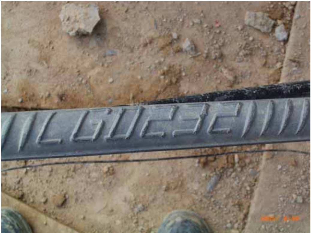
Figure 65: Bar mark was checked before grouting
