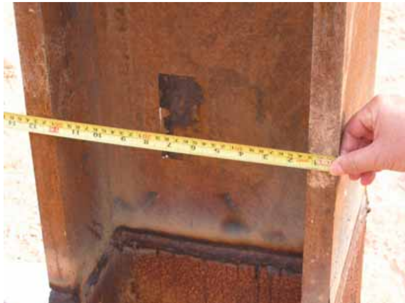
Figure 19: Dimension of pile was spot-checked by engineer
