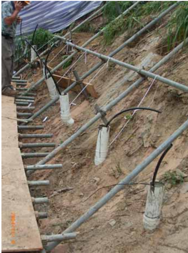
Figure 67: 300 mm pressure head is maintain after grouting
