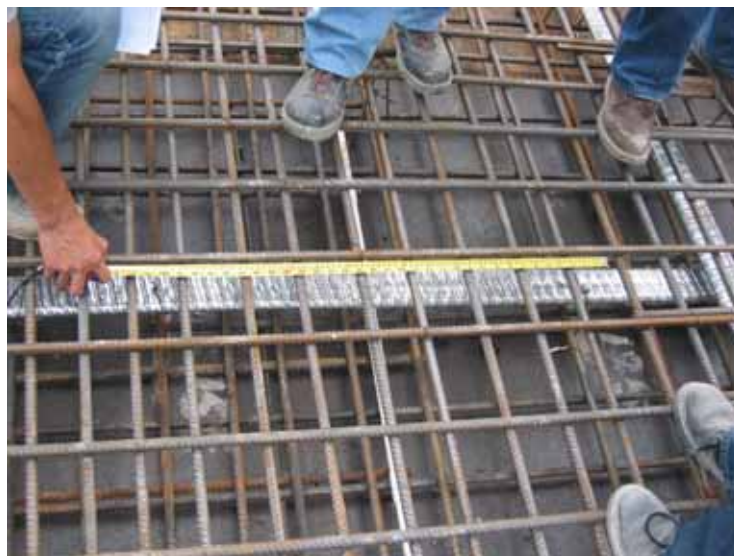
Figure 1: Prestress tendon is post-tensioning slab, Condition of tendon before concreting Pre-tensioning
