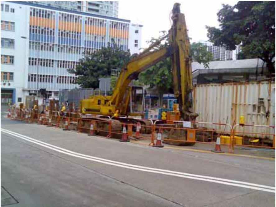
Figure 46: Backhoe was used in excavation works in drainage improve works.
