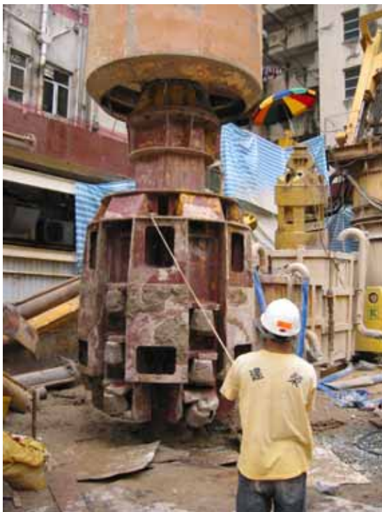
Figure 13: Machine used to construct the bell out
