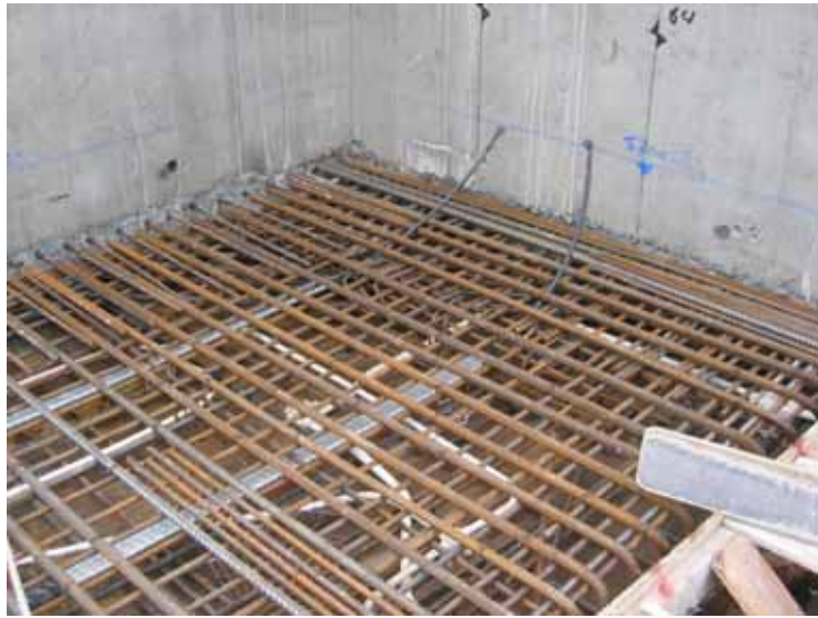
Figure 79: Reinforcement and other E&M parts checked before concreting
