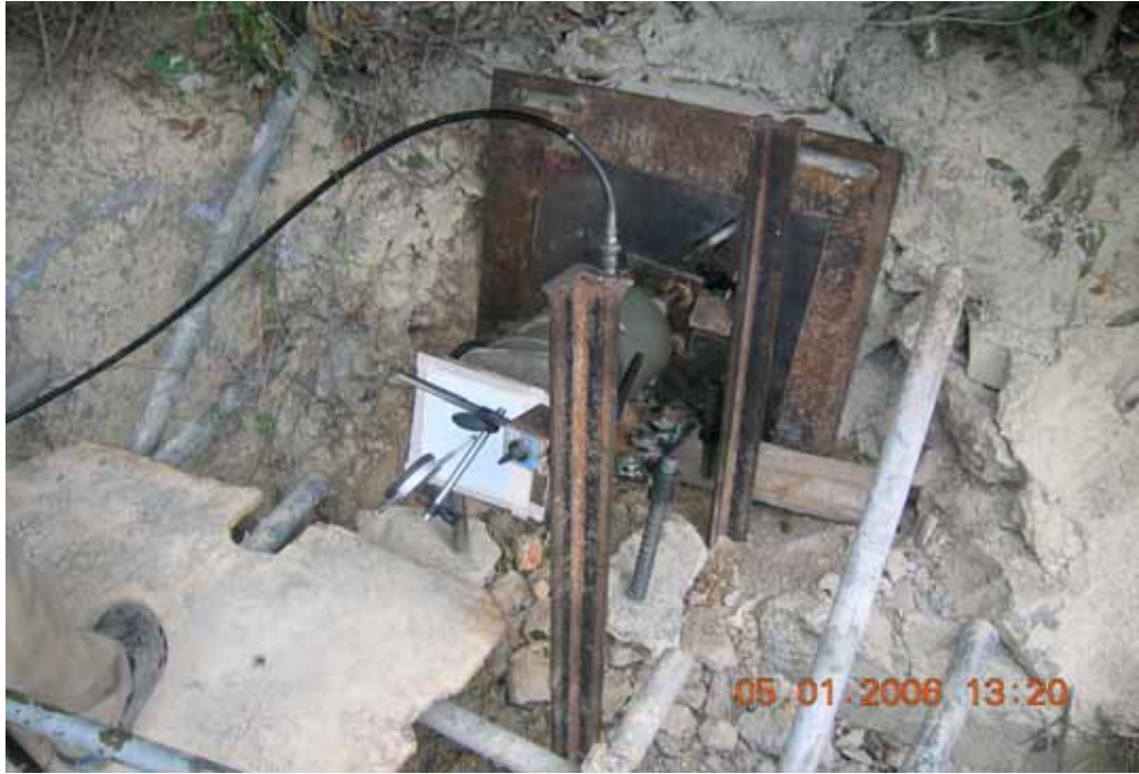
Figure 63: Pull out test in progress
