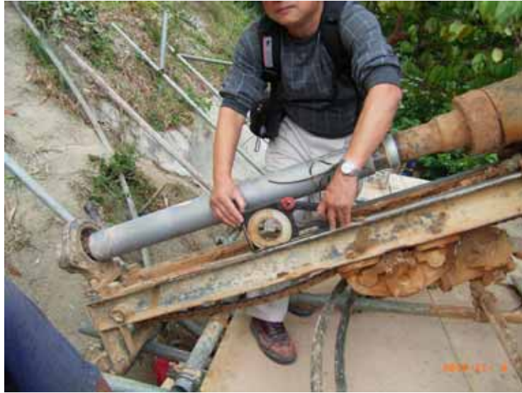
Figure 61: Engineer check the dip angle during drilling
