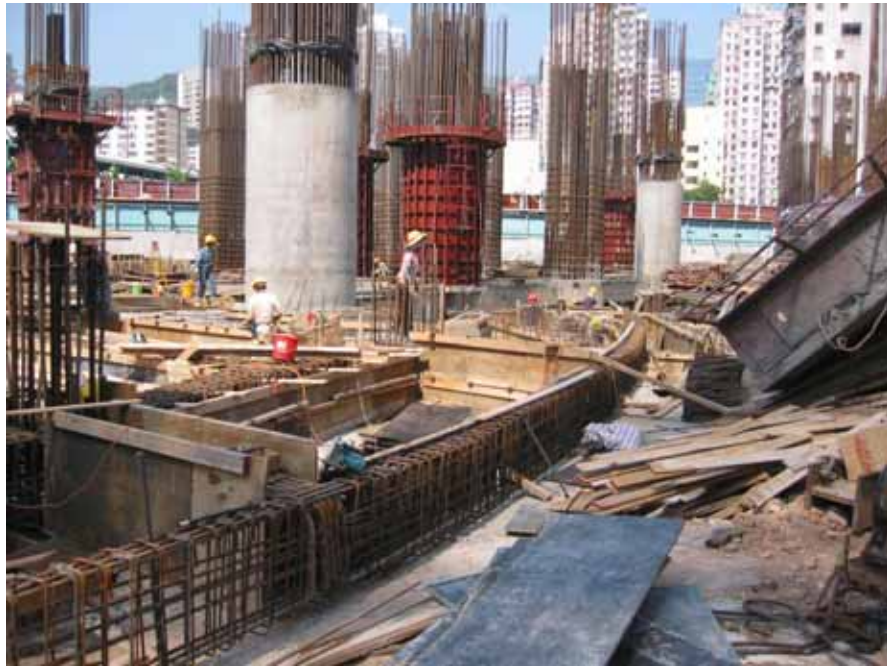
Figure 78: General view of column construction works
