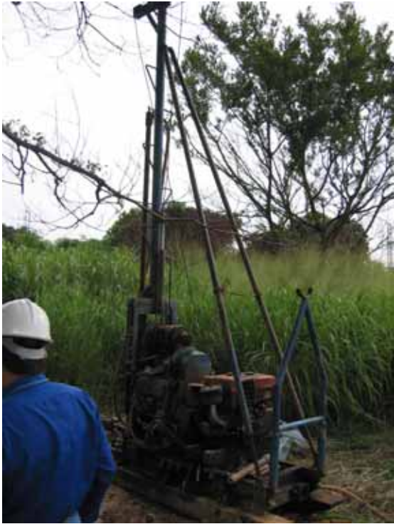
Figure 5: Drilling rig is used in drilling works
