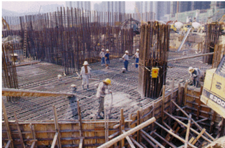
Figure 2: Concreting works for Pile Cap
