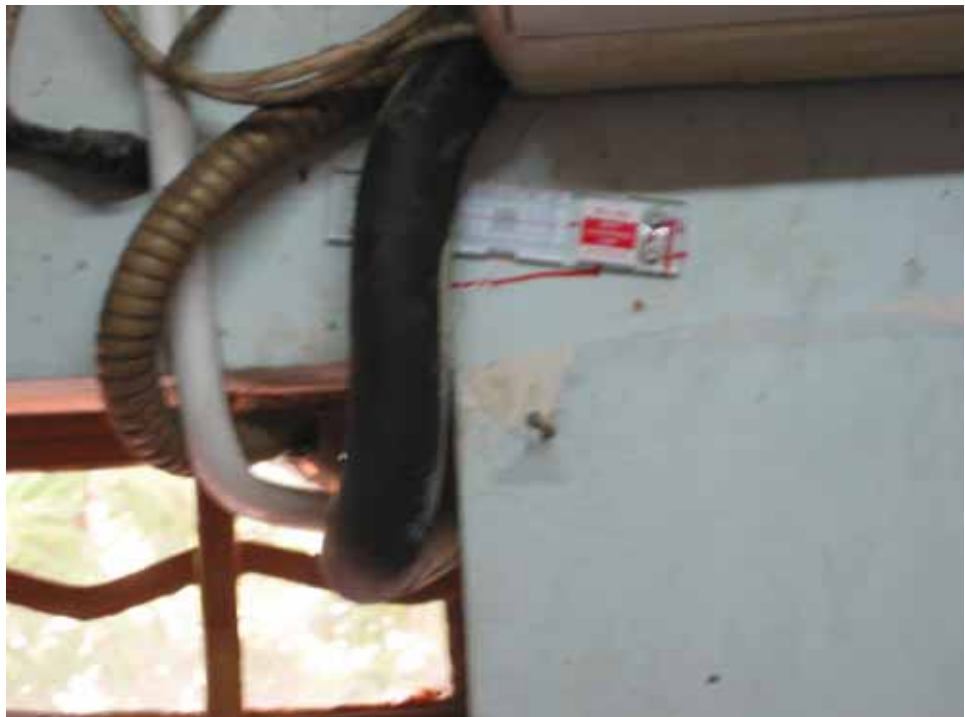
Figure 21: Tell-tale was used to check the movement of cracks
