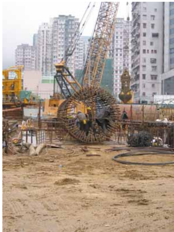
Figure 15: Reinforcement fixing for bored pile in progress
