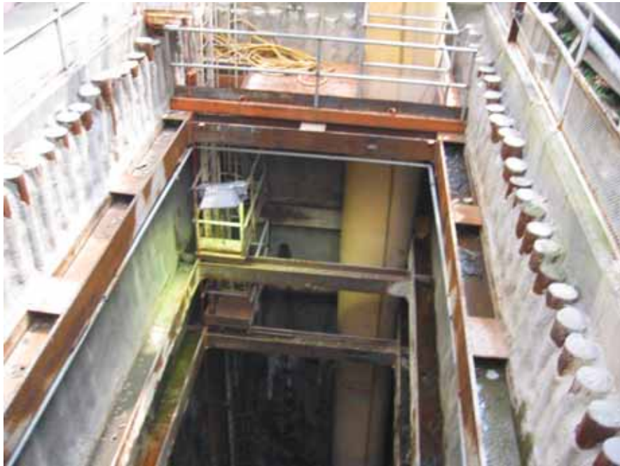
Figure 80: Pipe pile adopted as temporary retaining structure in excavation
