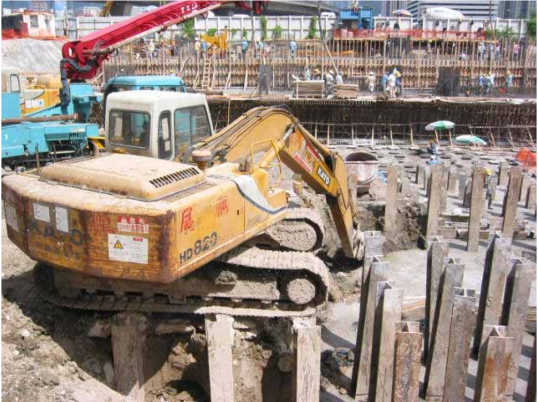
Figure 83: Backhoe was locate in a improper location to excavate the pile cap
