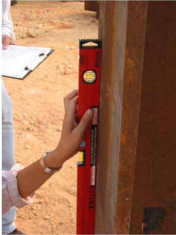
Figure 18: Verticality was checked during H-piling works
