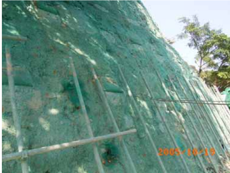
Figure 31: General condition of slope after hydro seeding
