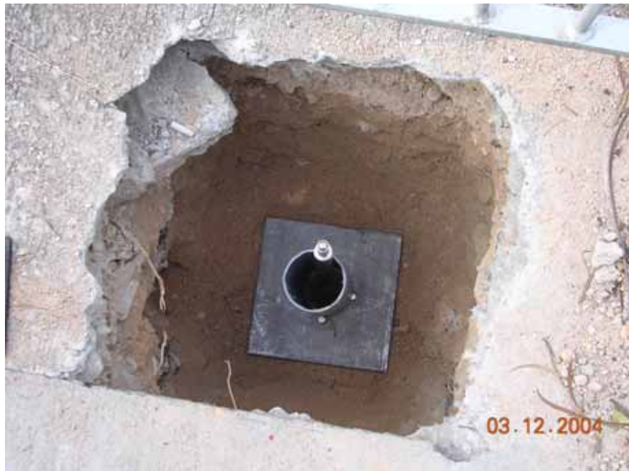
Figure 73: Settlement checkpoint was setup to check the settlement
