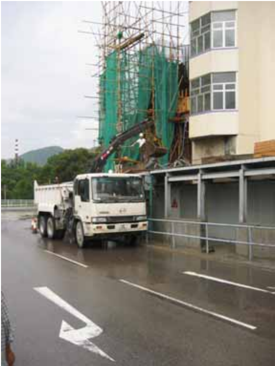
Figure 49: Grab lorry equipped with hydraulic rams and crane was used to deliver rubbish off site
