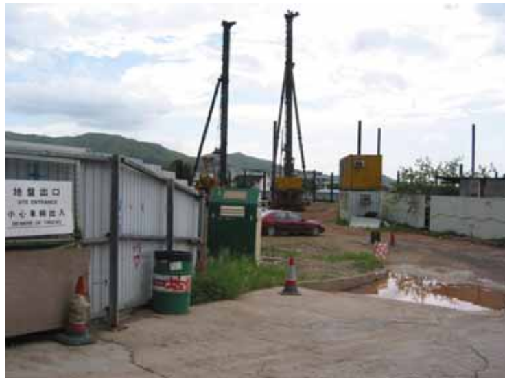
Figure 17: H-piling works in progress
