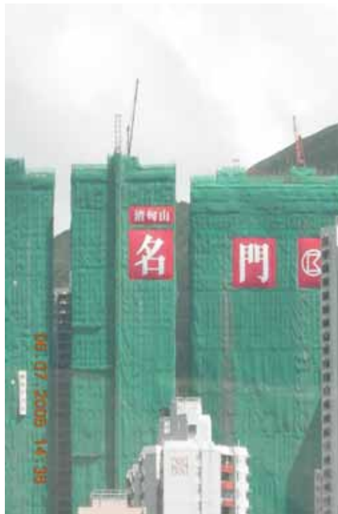
Figure 35: Bamboo scaffolding act as a safety mesh/ fence (precaution measure) in high-rise building
