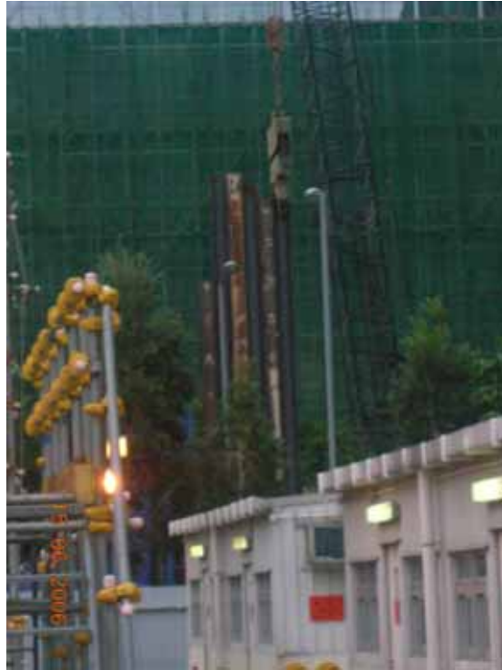
Figure 25: Sheet piling was installing by vibrating hammer
