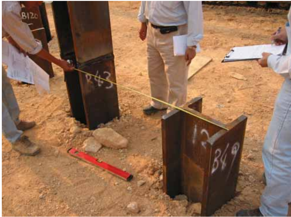
Figure 20: Setting out was checked by government
