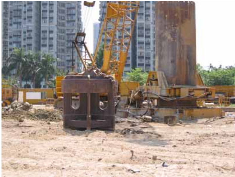
Figure 14: Chisel was used to overcome the boulder
