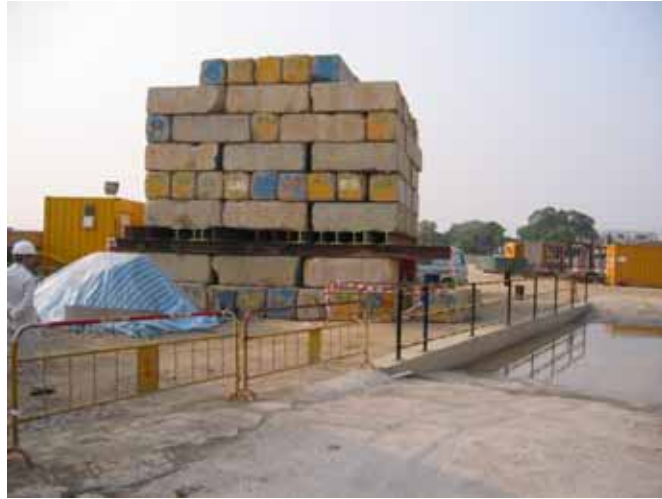
Figure 76: Loading test checking the pile
