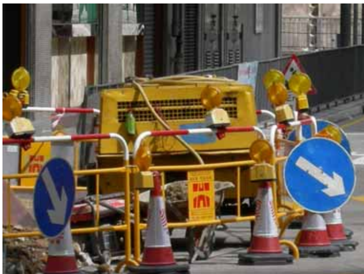
Figure 40: Air Compressor is used in road works to destroy existing concrete slab
