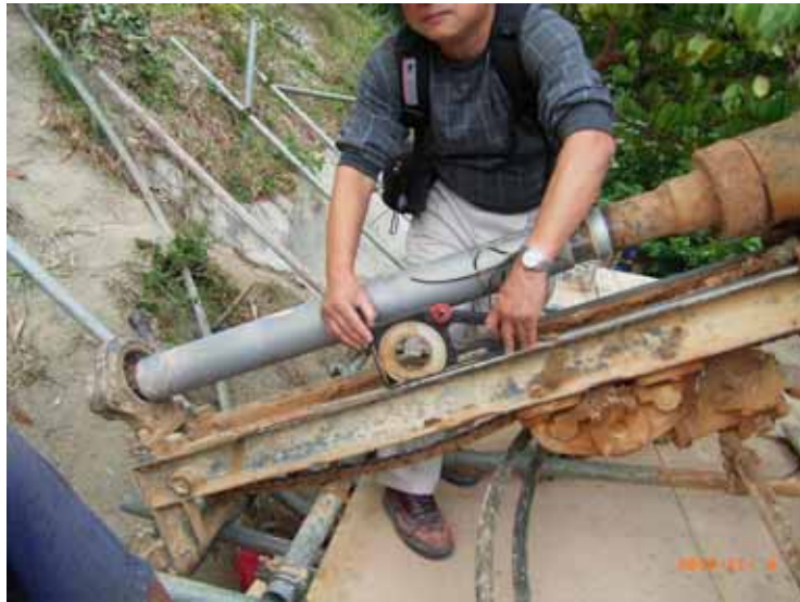
Figure 41: Drill rig used in soil nail works
