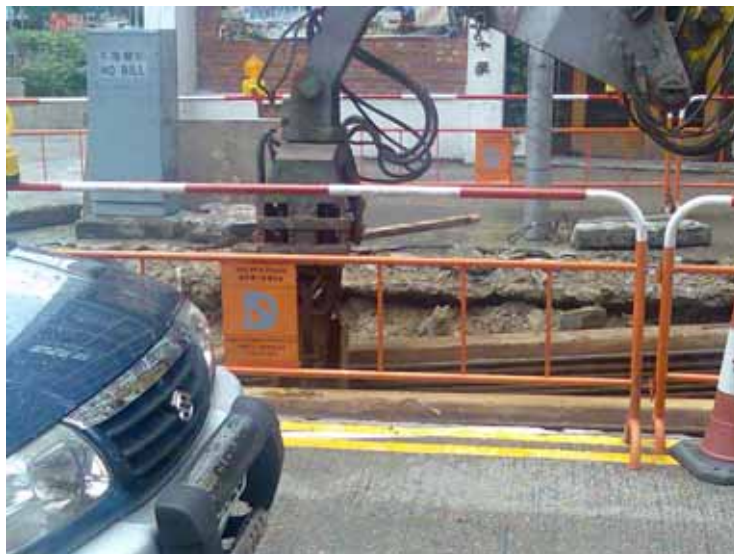
Figure 26: Sheet piling were installed to protect the existing road in drainage improve works
