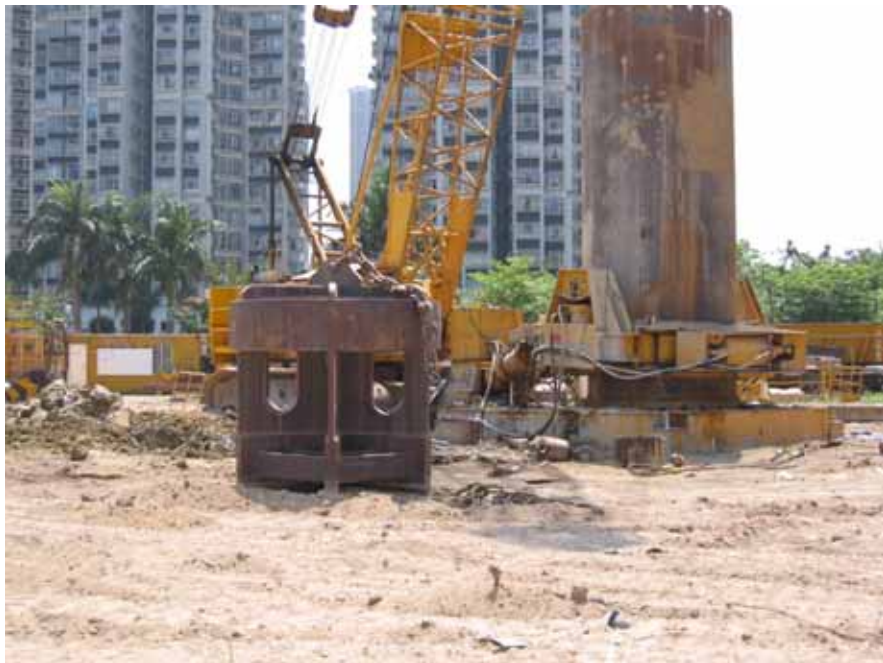
Figure 69: Chisel is used to overcome underground obstruction
