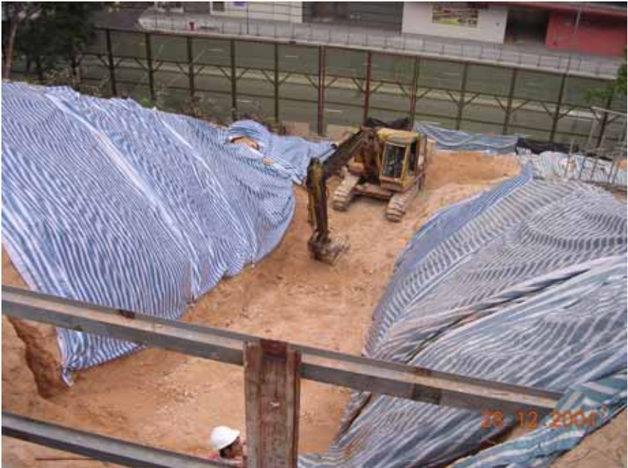
Figure 45: Backhoe was used in excavation works
