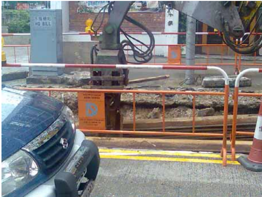
Figure 47: Backhoe was used in sheet piling installation.
