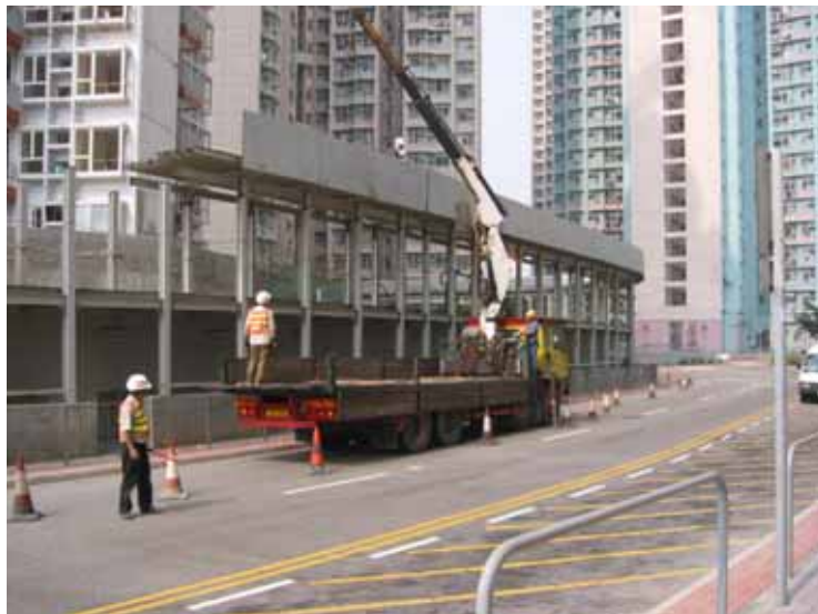
Figure 48: Crane Lorry was used to deliverer construction material
