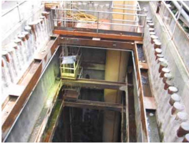
Figure 27: Pipe Pile Wall is used to support existing buildings in shaft excavation
