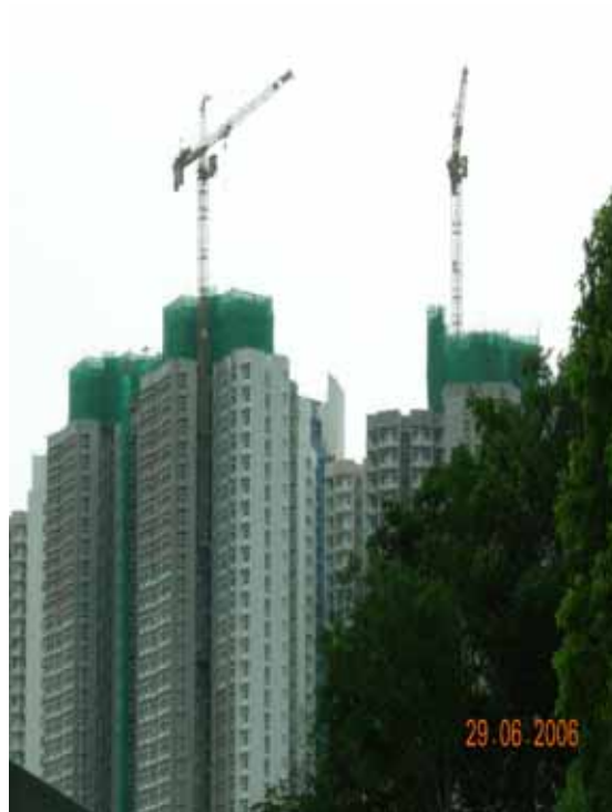
Figure 42: External climbing Tower Crane
