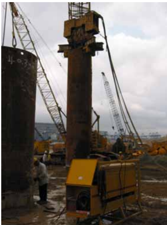
Figure 12: Vibro hammer is used to insert the steel casting
