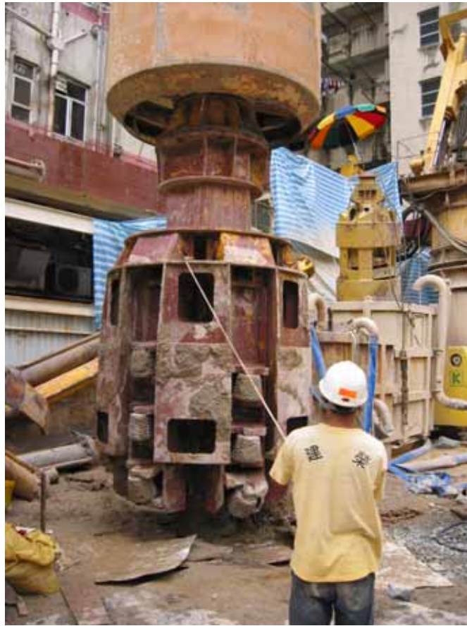
Figure 70: Belling tools used to construct the bell out of bored pile
