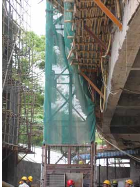
Figure 55: Material hoist was used in construction site
