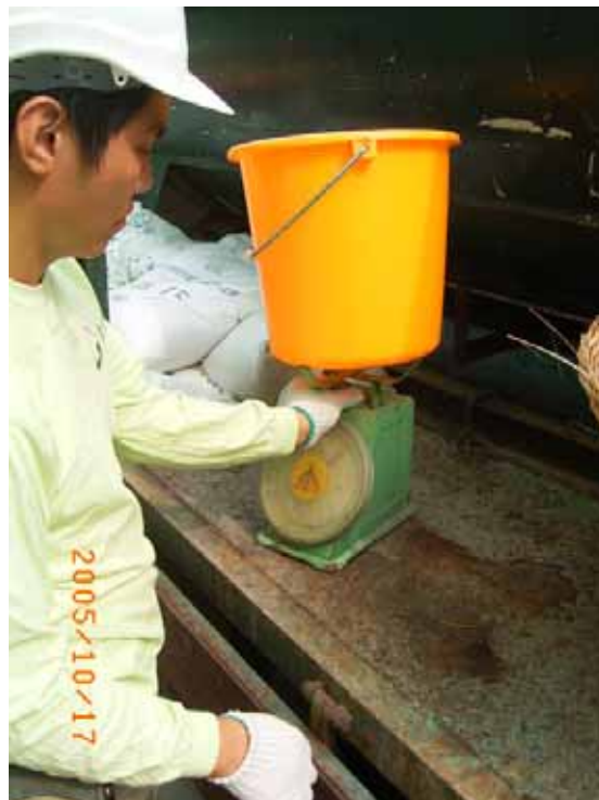
Figure 30: Weight of the grass seed was measured before hydro seeding
