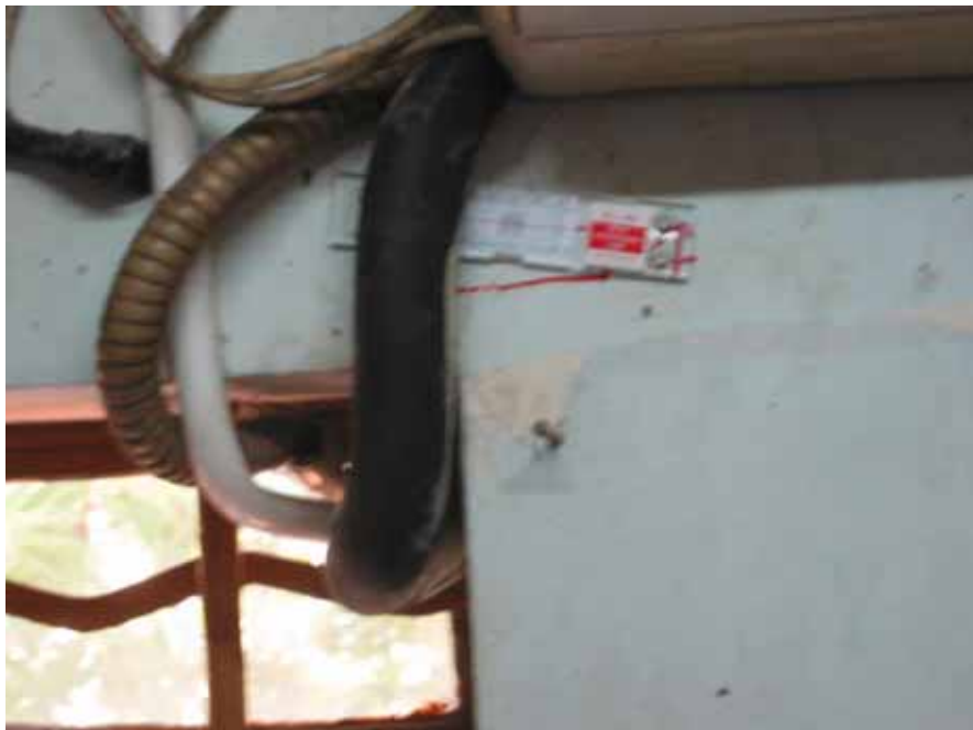
Figure 75: Tell-tale adopted to monitor the width of crack
