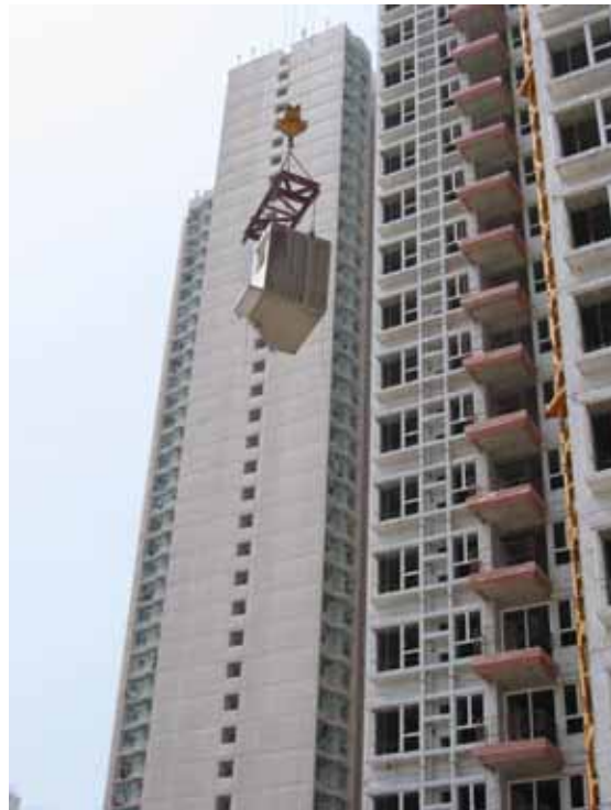
Figure 34: Pre-cast façade before installation
