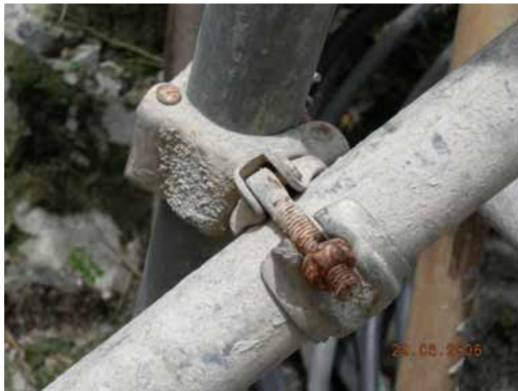
Figure 37: Coupler used in metal scaffolding
