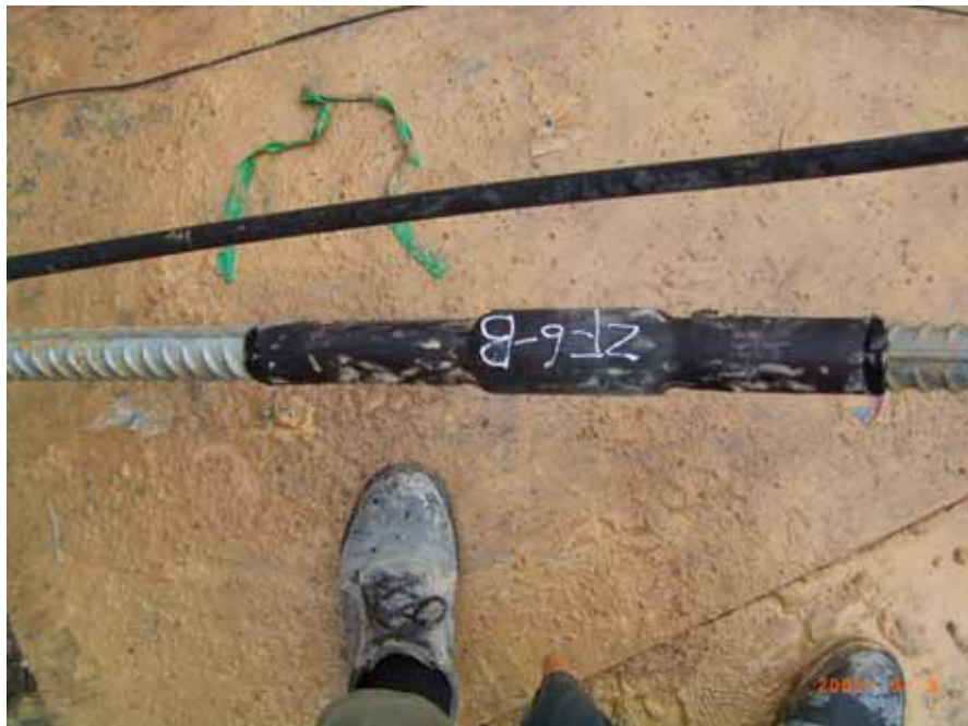
Figure 66: Heat-shrinking sleeve is used protect the coupler
