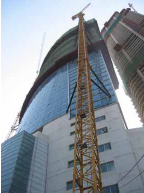
Figure 43: Tower Crane was used in circular-shaped building Concrete Pump
