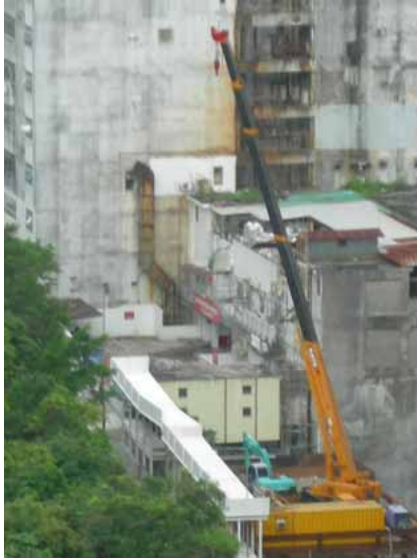
Figure 57: A typical mobile crane with telescopic jib
