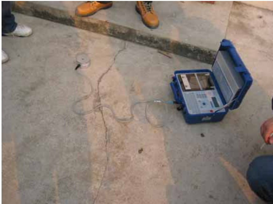
Figure 74: Monitoring the vibration during H-pile Construction Works
