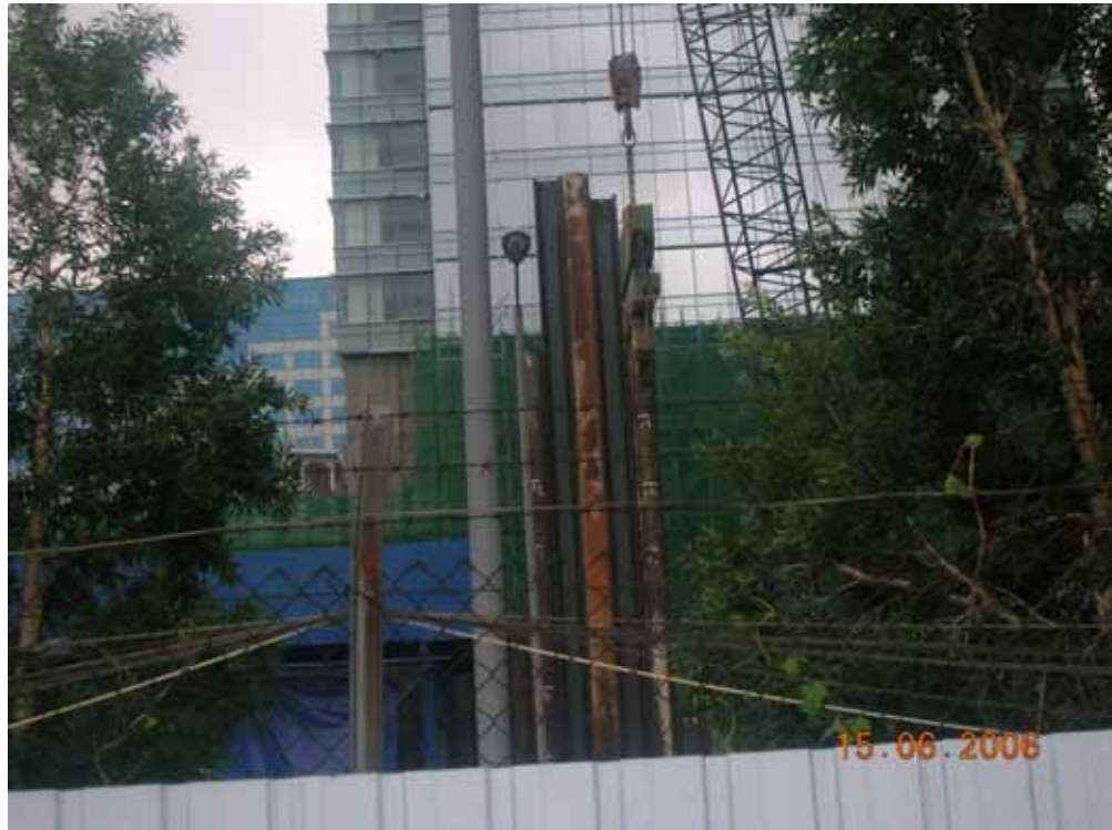
Figure 82: Steel Sheet Piling was installed as temporary works in excavation
