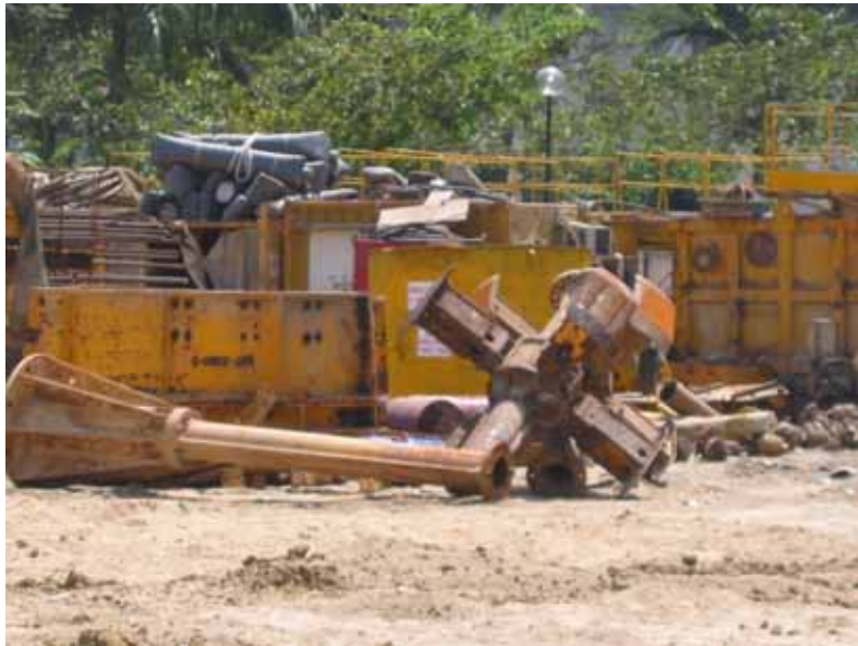
Figure 10: Equipment is used to ensure the drilling rig vertical
