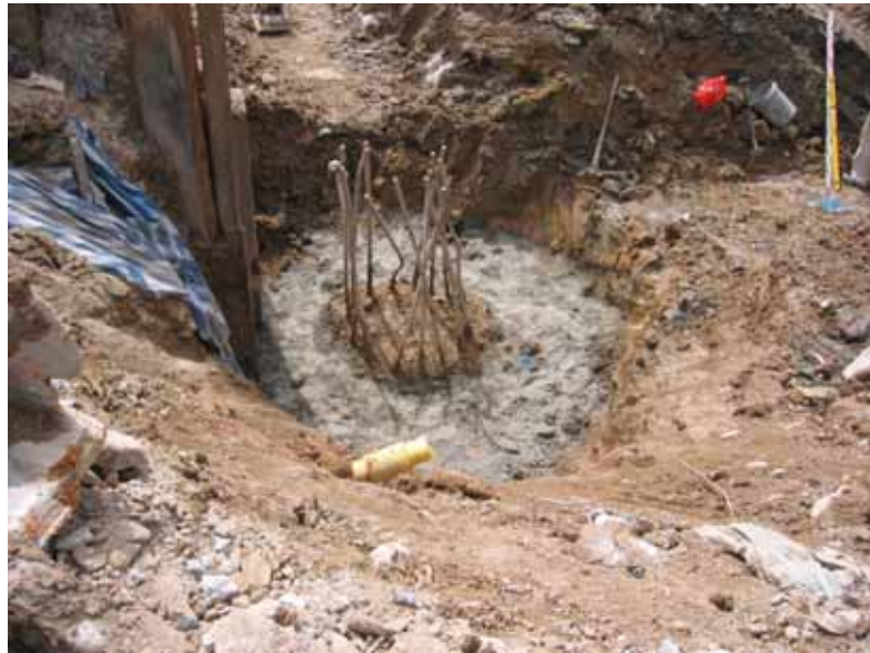
Figure 16: Excavation works for pile cap and cut-off
