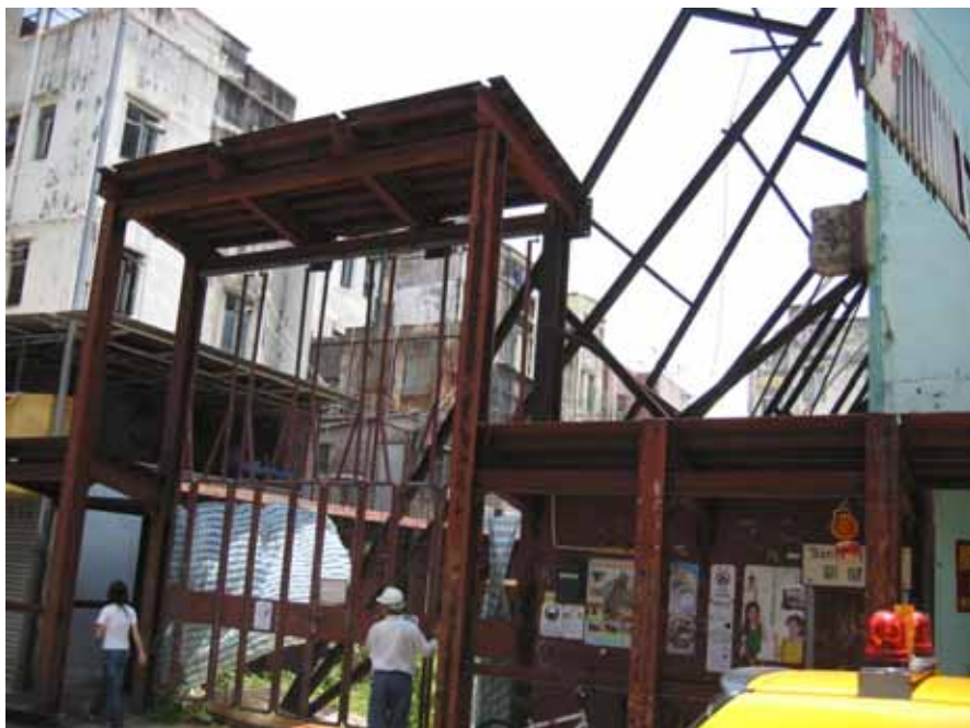
Figure 23: Shoring was provided to support adjacent building
