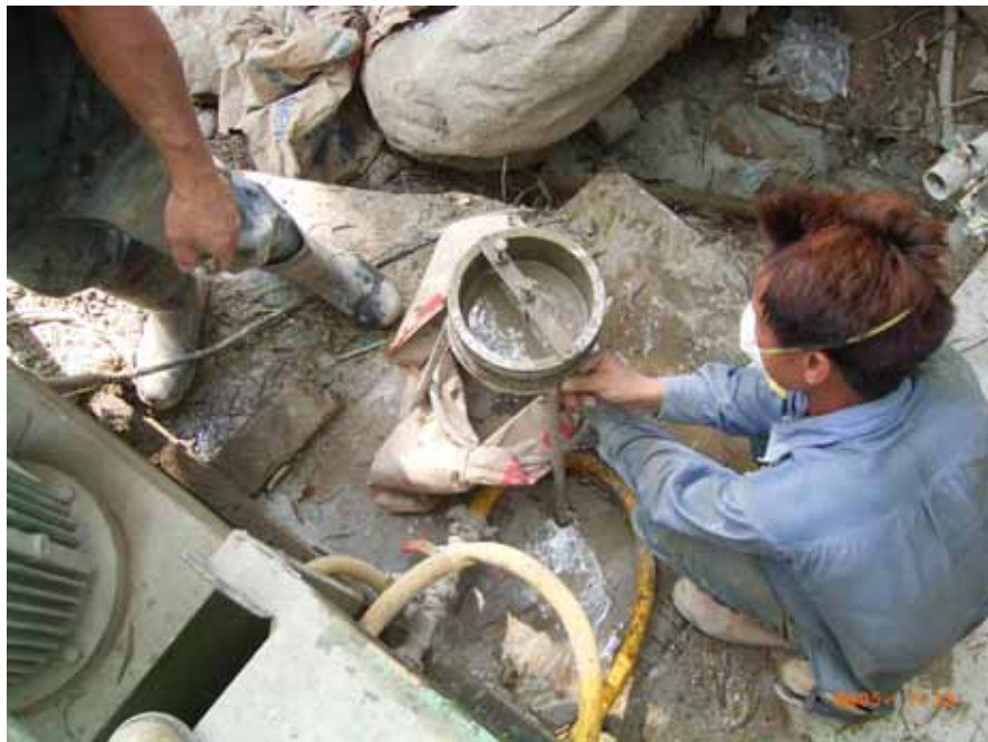
Figure 71: Flow cone test to check the workability of cement grout
