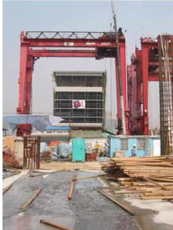
Figure 50: Gantry Crane was used to lift up heavy object
