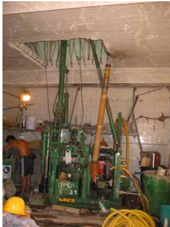
Figure 8: Mini-pile was used because of headroom limit Odex method is used in mini-pile construction works
