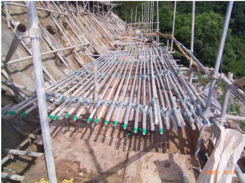
Figure 64: Soil nail bar before grouting
