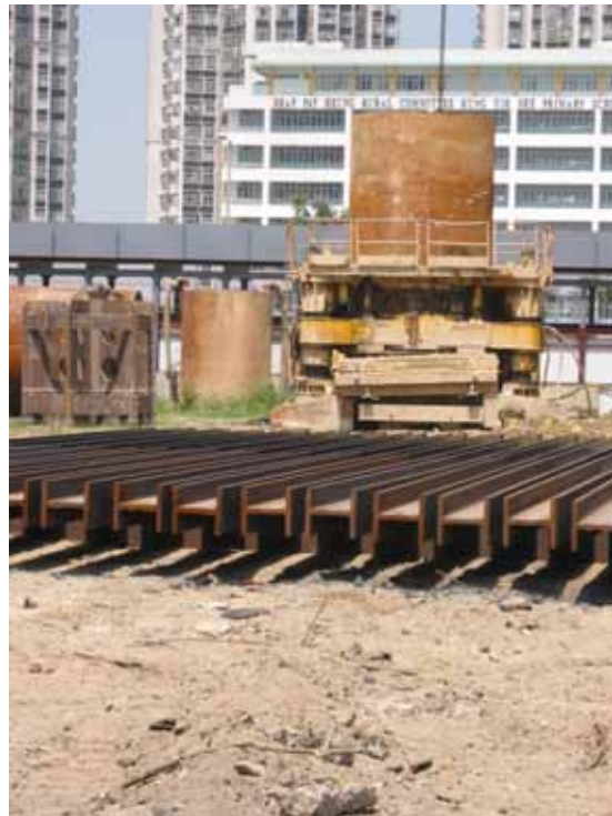
Figure 9: Steel casting is used in bored pile works
