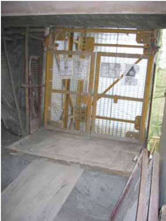
Figure 54: Passenger hoist entry at high
