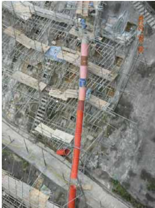
Figure 51: Rubbish Chute was used to deliver Rubbish from High
